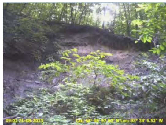
Side hill seeps cause slope instability
