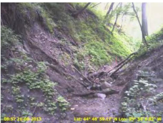
Loss of channel bottom and toe erosion cause slope failure
