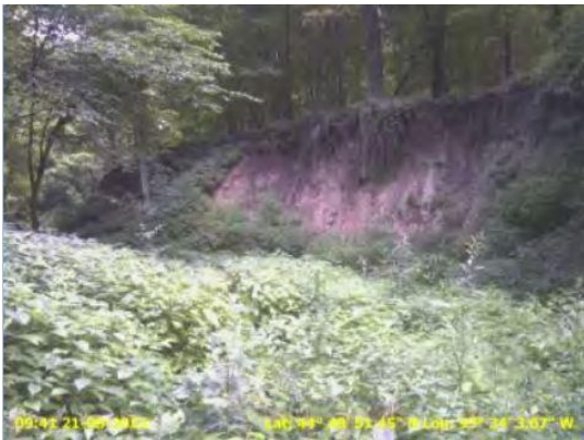
Channel migrating to the steep bluff slope and a loss of access to the floodplain has caused toe erosion and slope failure.
