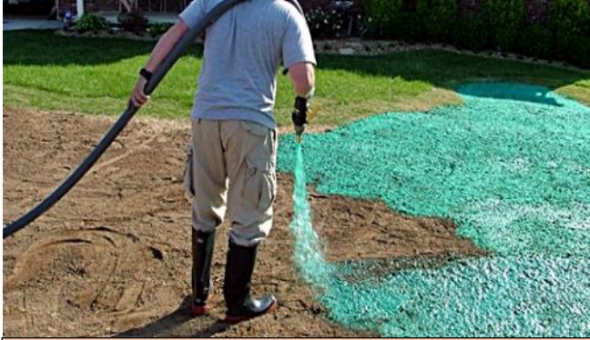
Image 2- 49: Hydroseeding. At this site you can clearly see the soil was raked and smoothed in preparation for the hydromulch (photo: clarkslandscape.com).
