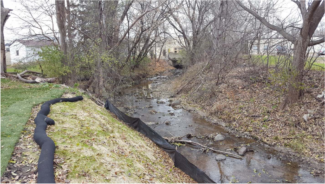
Photo 6: Site M9 – debris in channel upstream of site repaired by city of Chaska
