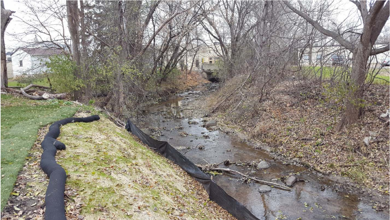
Photo 18: Site S7 – recent repairs made by city of Chaska
