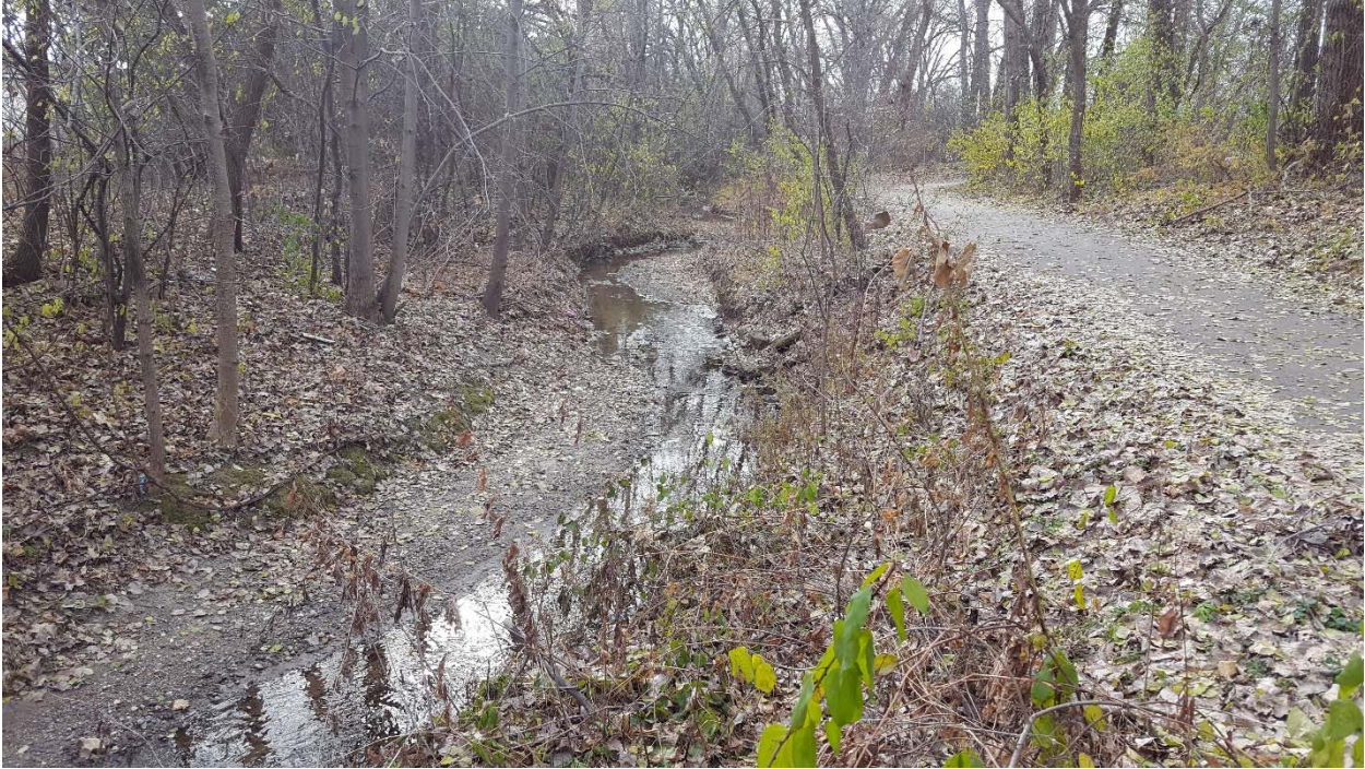
Photo 3: Site M6 – bank erosion adjacent to a PVC outfall
