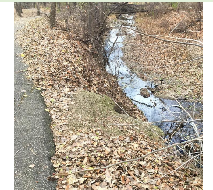
Nov. 2018 Field Visit: Eroded eastern bank – in both images (2016 and 2018) the light gray coloring is concrete installed to mitigate loss of bank.
