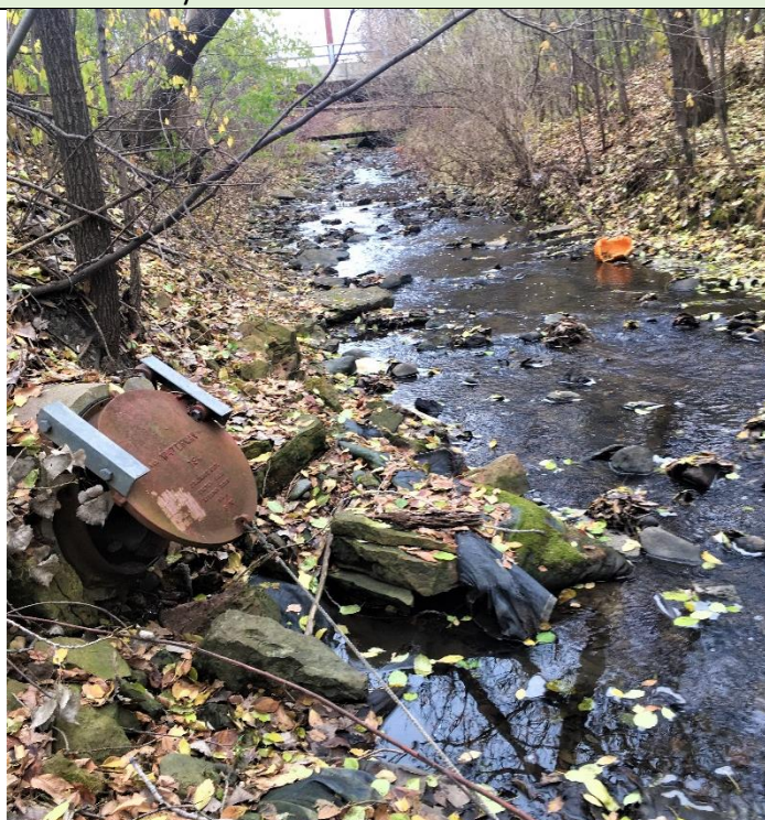
Nov. 2018 Field Visit: Upstream (western) view of RCP outlet.
