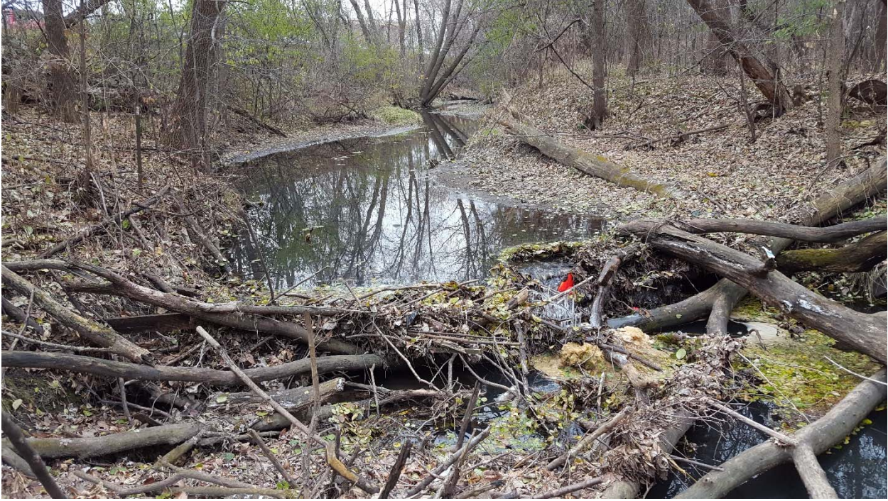
Photo 9: Site M12 – debris jam causing blockage and backwater
