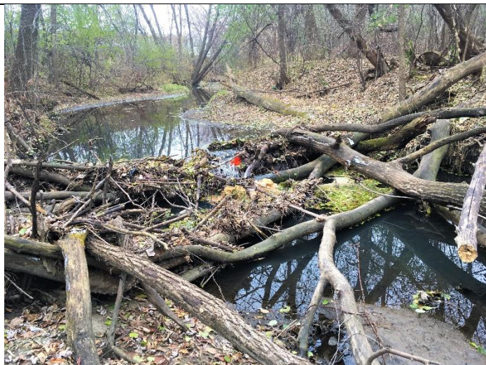
Nov. 2018 Field Visit: Debris downstream of levee, near Carver County Courthouse.
