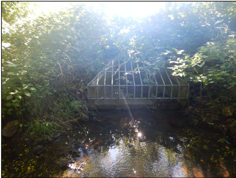
Photograph A-1: View east of RCP outfall.
