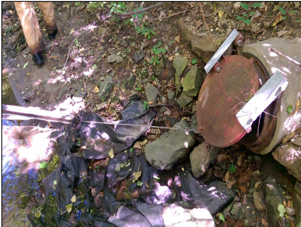
Photograph A-12: View east of RCP outlet.
