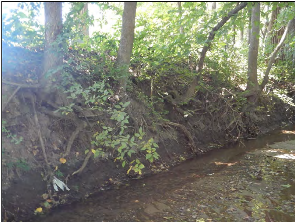
Photograph B-12: View south of eroded bank.
