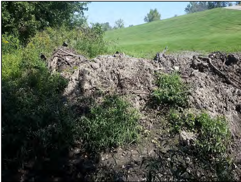
Photograph C-4: View north of potential settling basin.
