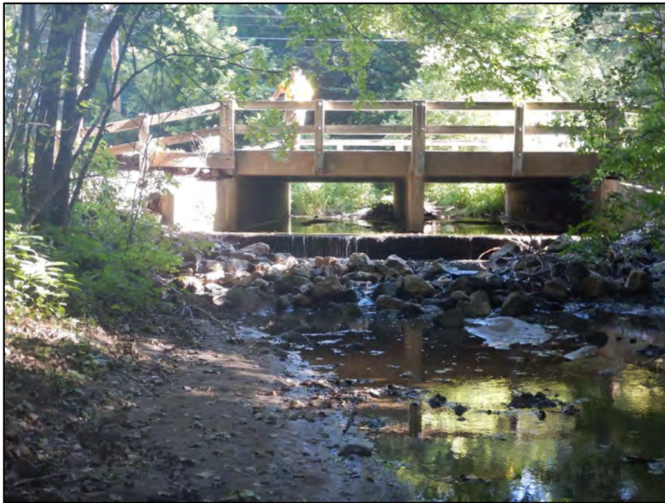
Photograph B-2: View northeast of bridge crossing.
