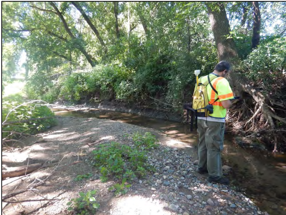
Photograph B-14: View south of eroded bank.
