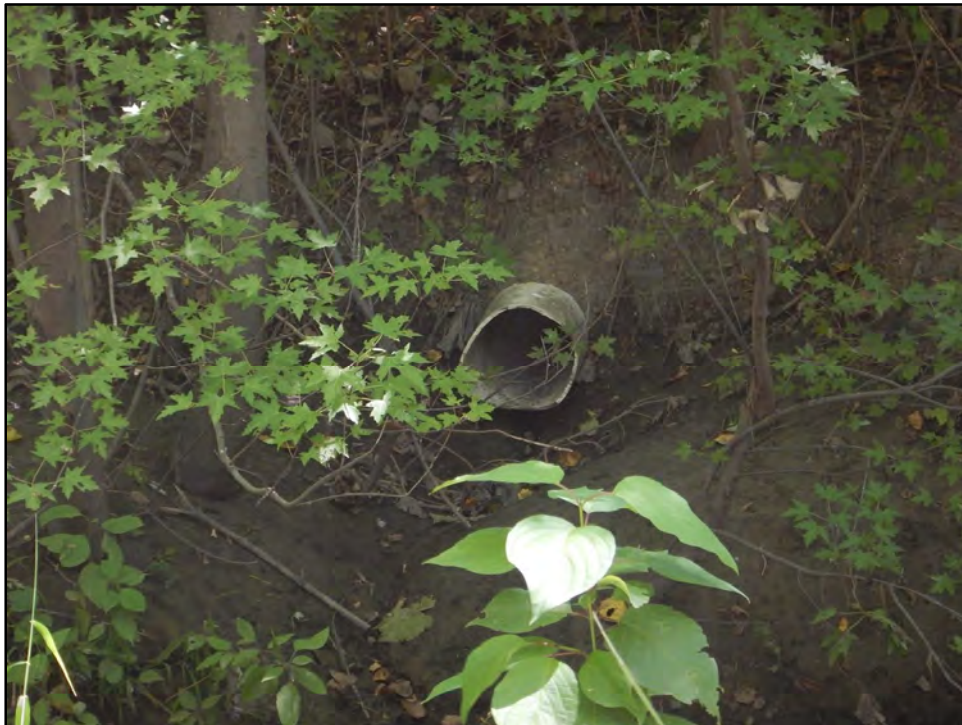
Photograph A-6: View east of PVC outfall.
