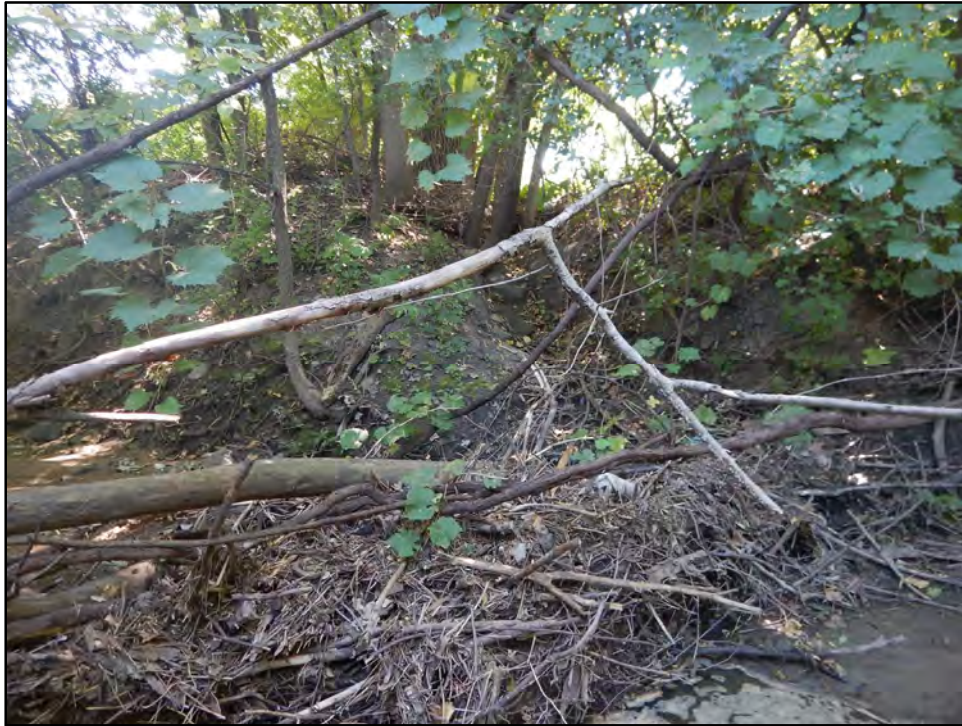
Photograph A-10: View east of debris.
