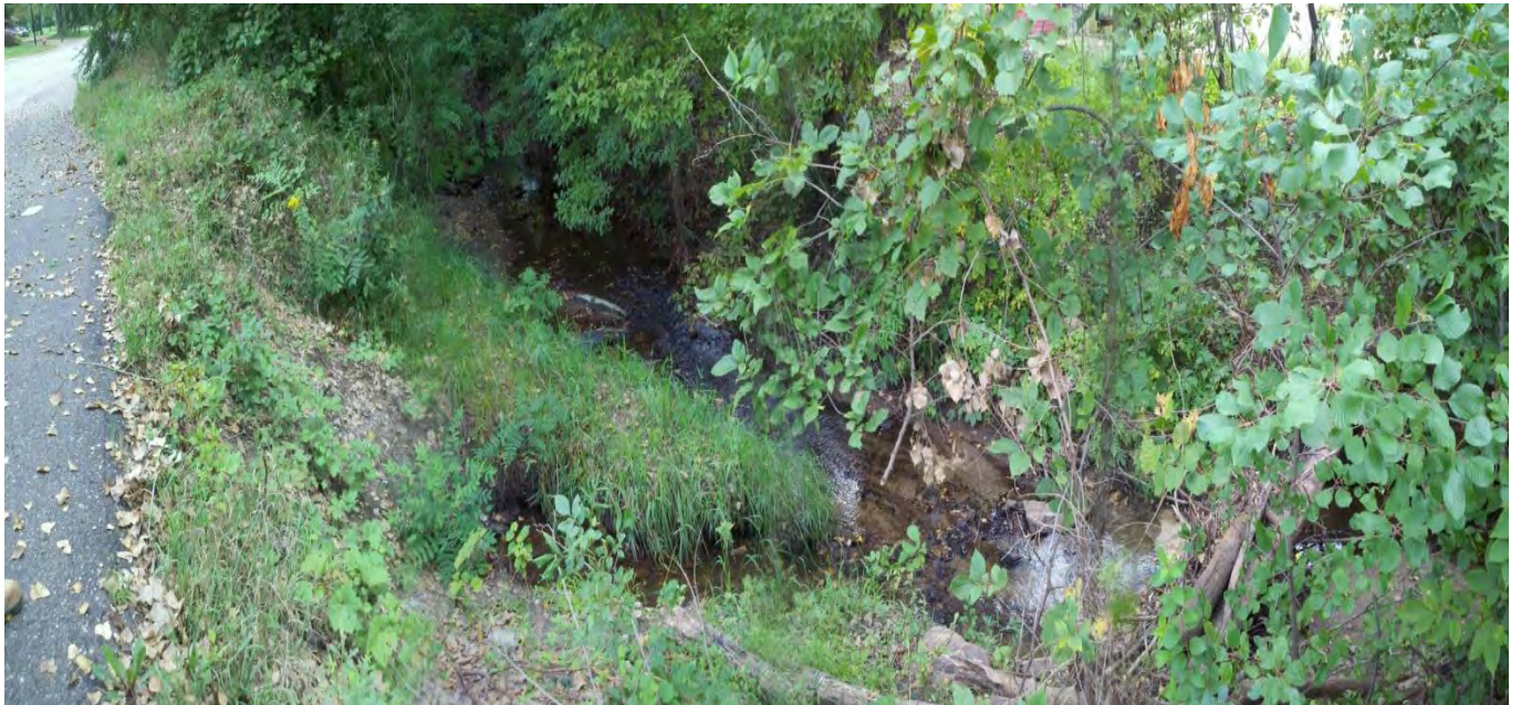
Photo 8. East Chaska Creek Outfall A (just downstream of Arby's parking lot)
