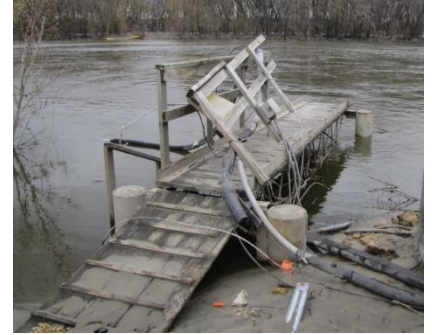
Flood damage, sensor lost 2011
