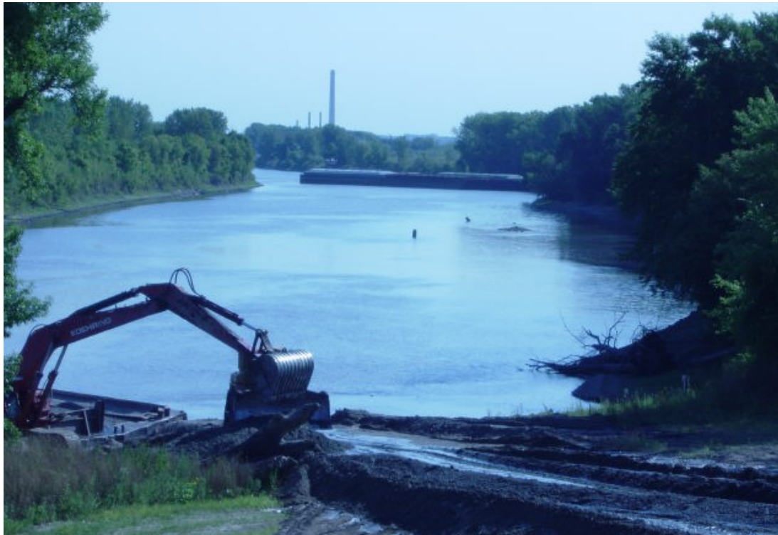
Dredging operations at Savage
