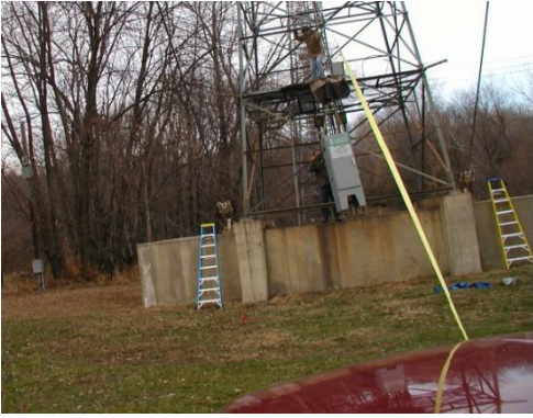
Gage installation, Oct. 2003
