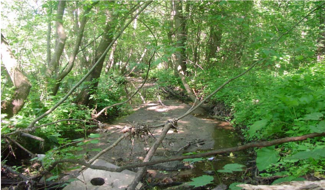
Channel upstream of RR crossing showing scour from storm sewer discharges
