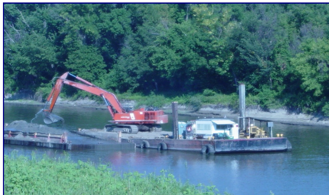
Minnesota River dredging in-process by the U.S. Army Corp of Engineers
