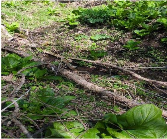
Photo 2. BLM151 Gully Condition
