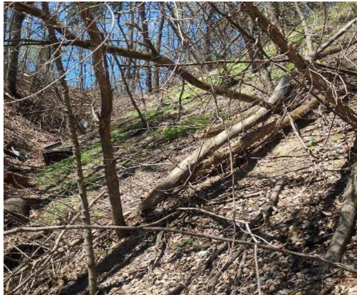
Photo 1. CVR63 Gully Condition
