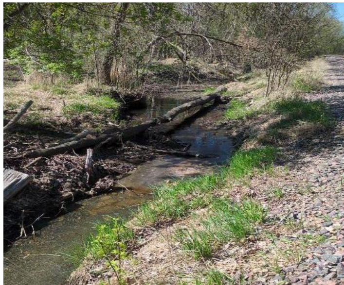
Photo 5. BVL52 Gully Condition
