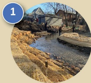
1 Spring Creek Site Stabilization
