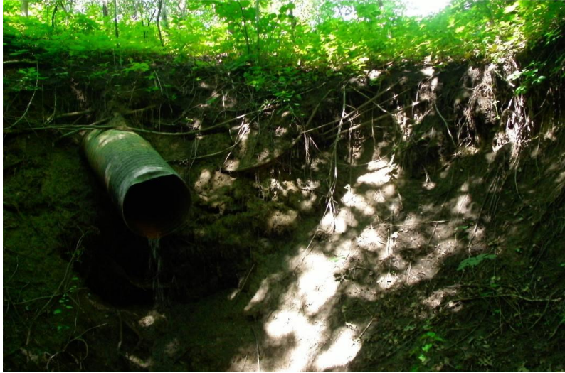
Tile drainage outlets can form plunge pools at the head of ravines.
