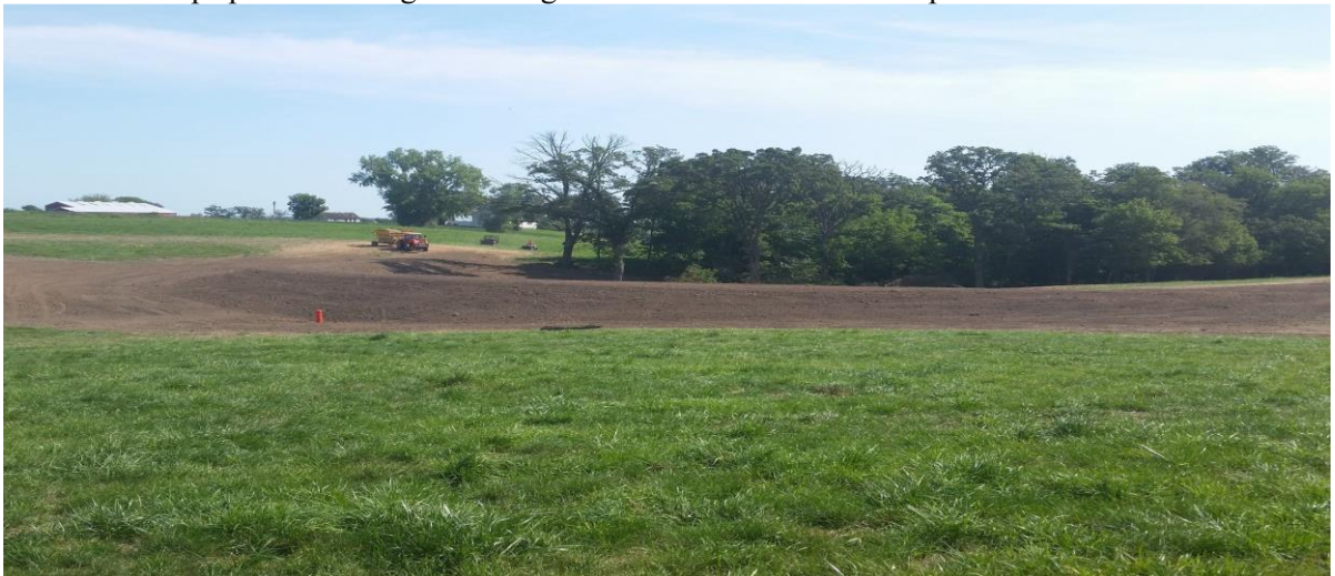
Constructed WASCOB at head of ravine, Goodhue County SWCD
