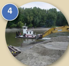
4 Vernon Avenue Dredge Material Management Site
