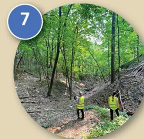
7 Gully Inventory and Condition Assessment - Phase 3
