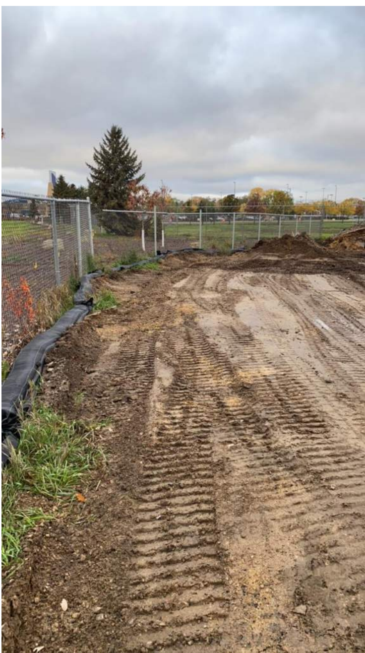
Perimeter sediment control BMPs on Project site
