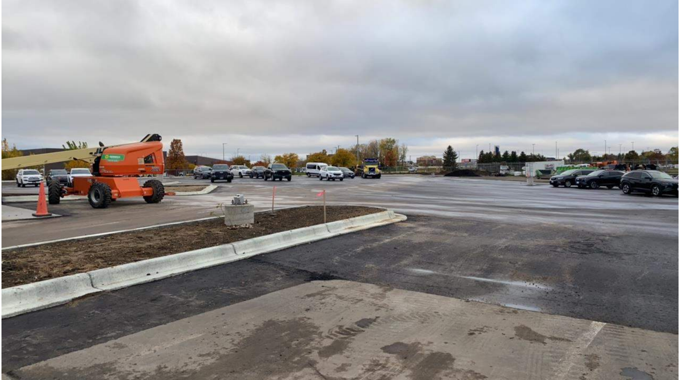
Impervious surfaces completed in the correct locations as shown on plans
