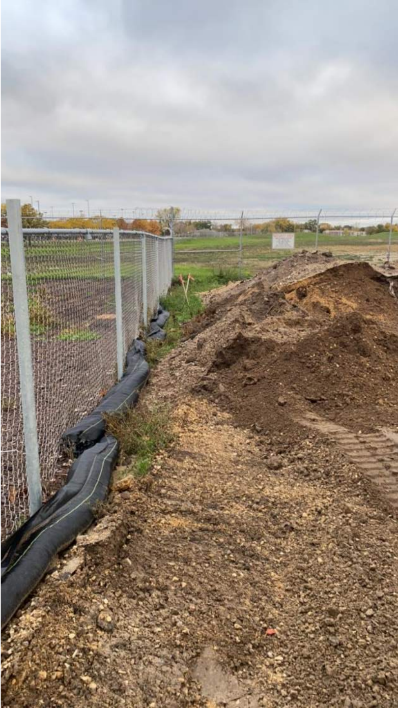
Stockpile with temporary BMPs surrounding
