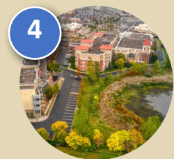
4 City of Shakopee Downtown Stormwater Best Management Practices (BMP) (see page 6)
