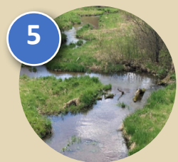
5 Eagle Creek Bank Stabilization (see page 6)
