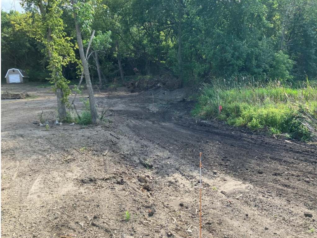
Photo 5: fill removal at 5250 Eagle Creek Blvd, Shakopee
