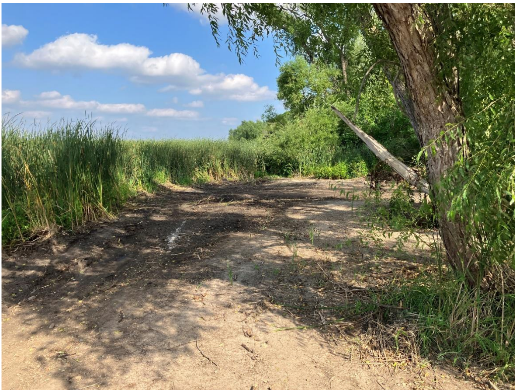
Photo 6: fill removal at 5250 Eagle Creek Blvd, Shakopee
