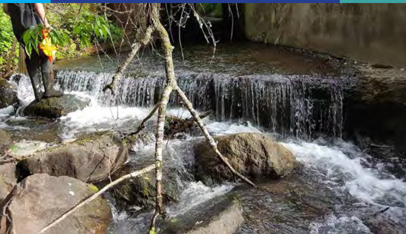
Scouring on the downstream side of Flying Cloud Drive is representative of active erosion in Riley Creek
