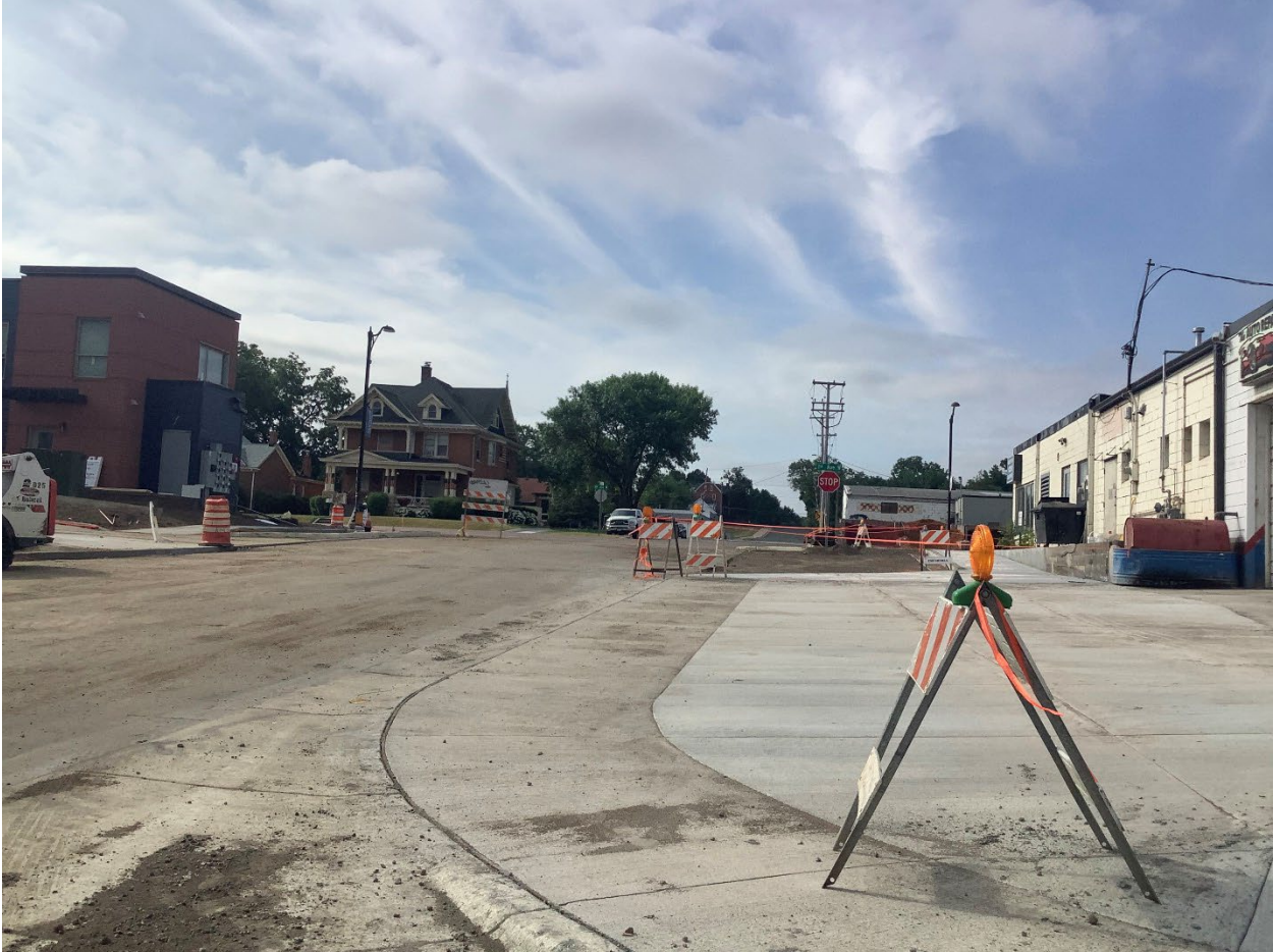
Figure 3. Current construction on Scott St
