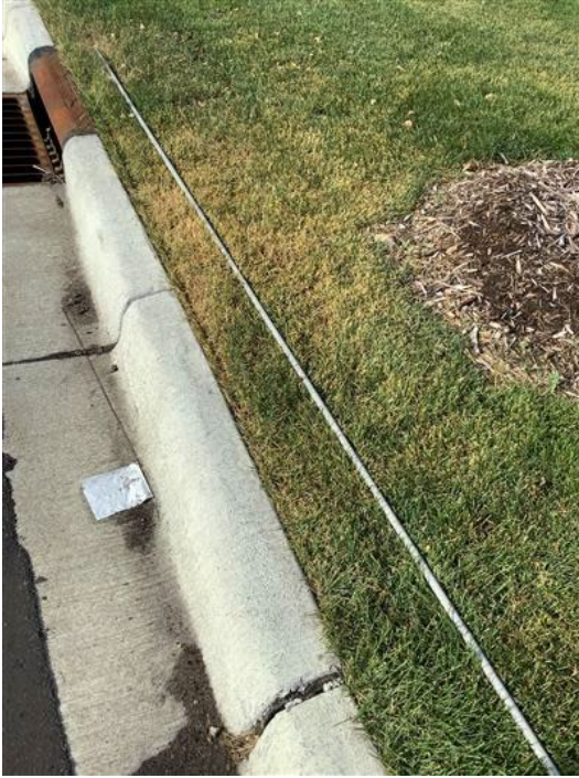
Figure 3—Pole found on southwest corner of site.
