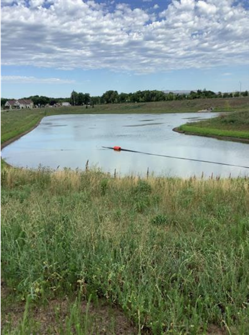
Figure 1. Silt curtain in pond
