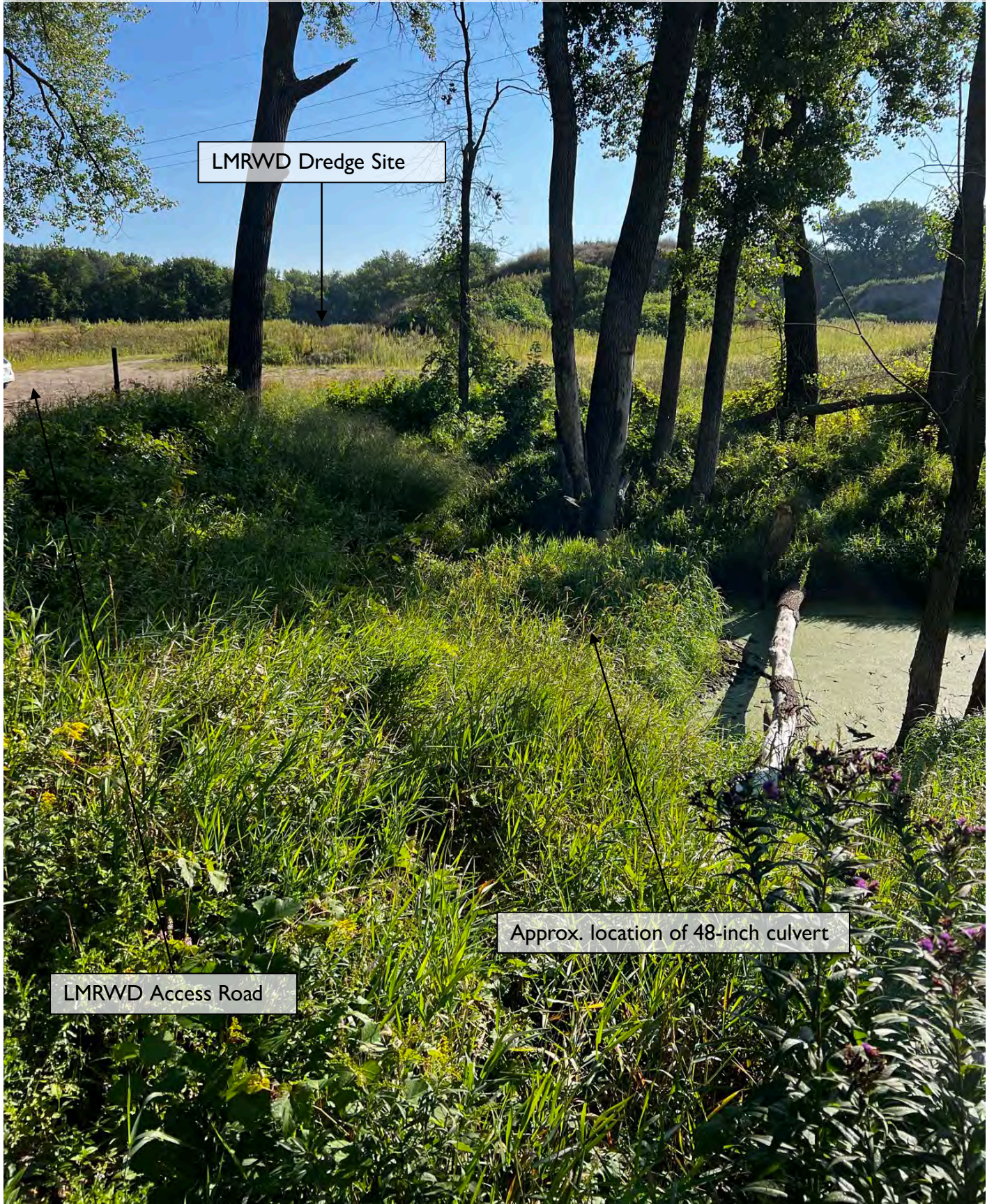
Photo 1A. LMRWD Dredge Site access road culvert (upstream, not visible due to dense vegetation)
