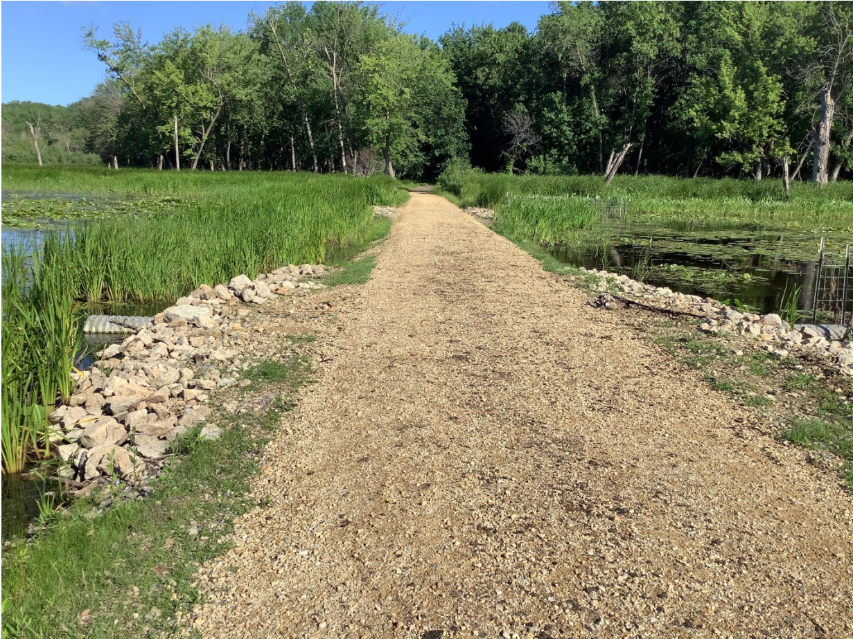
Figure 1. South culvert replacement area
