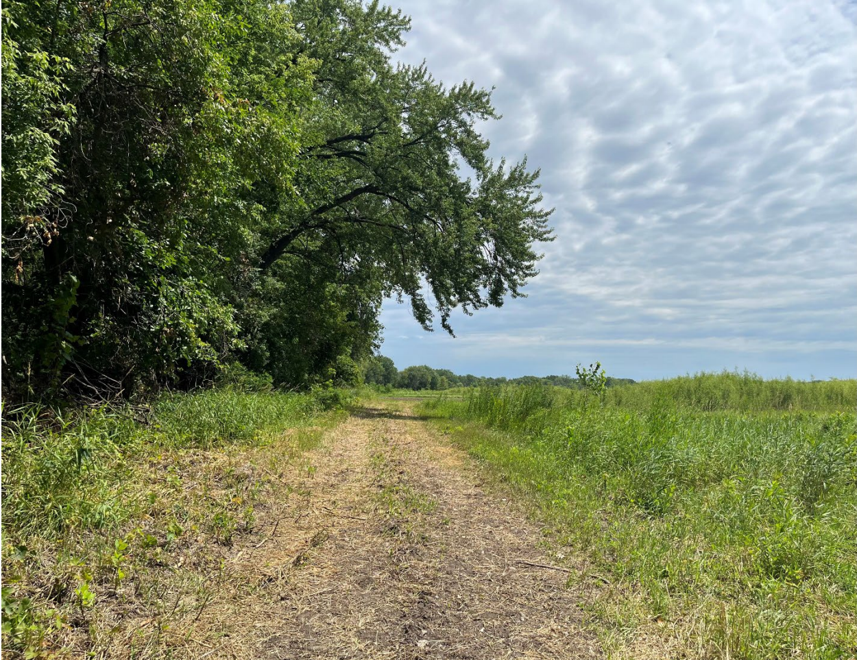
Figure 5. Road maintained looking east
