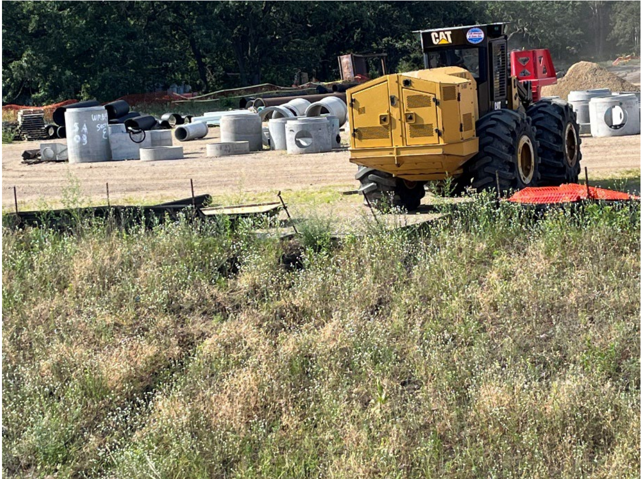
Figure 1. Falling silt fence
