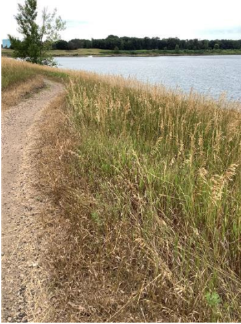
Figure 2. Erosion control blanket (east side of site)
