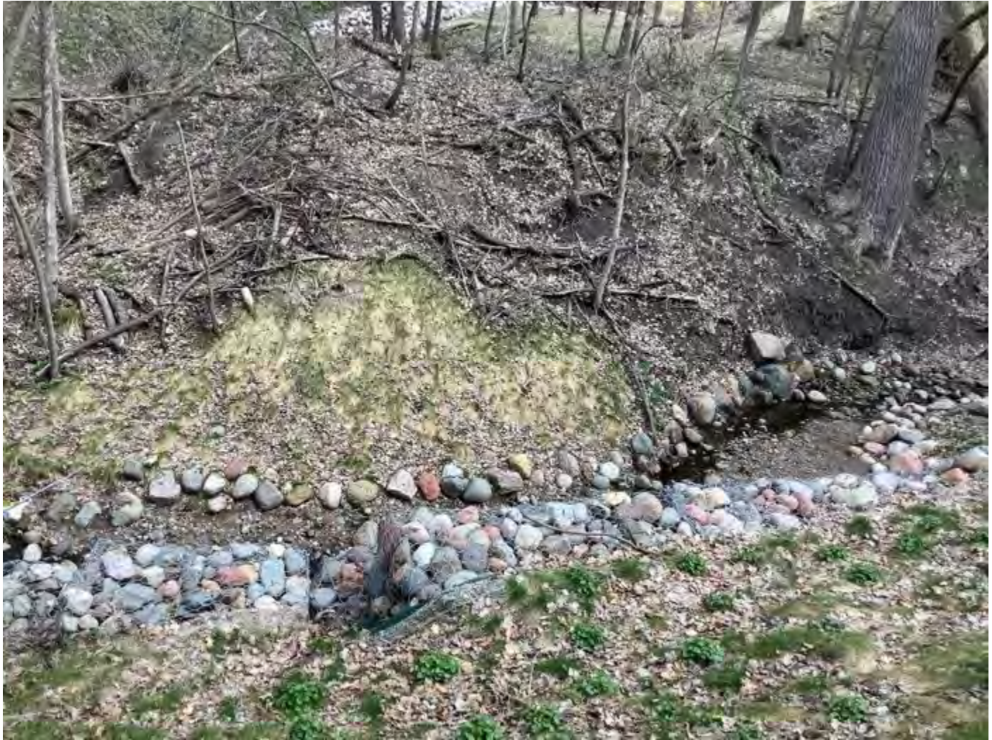
Erosion control structures
