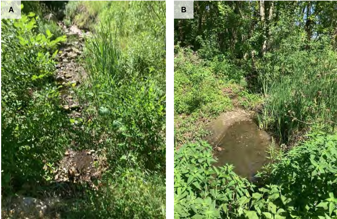
Figure 22. Photos of Gully 06:15-10:13. A) Upstream view of south side of trail. Severe degradation is visible on the left bank upstream. B) Downstream view of north side of trail of gully with stagnant water
