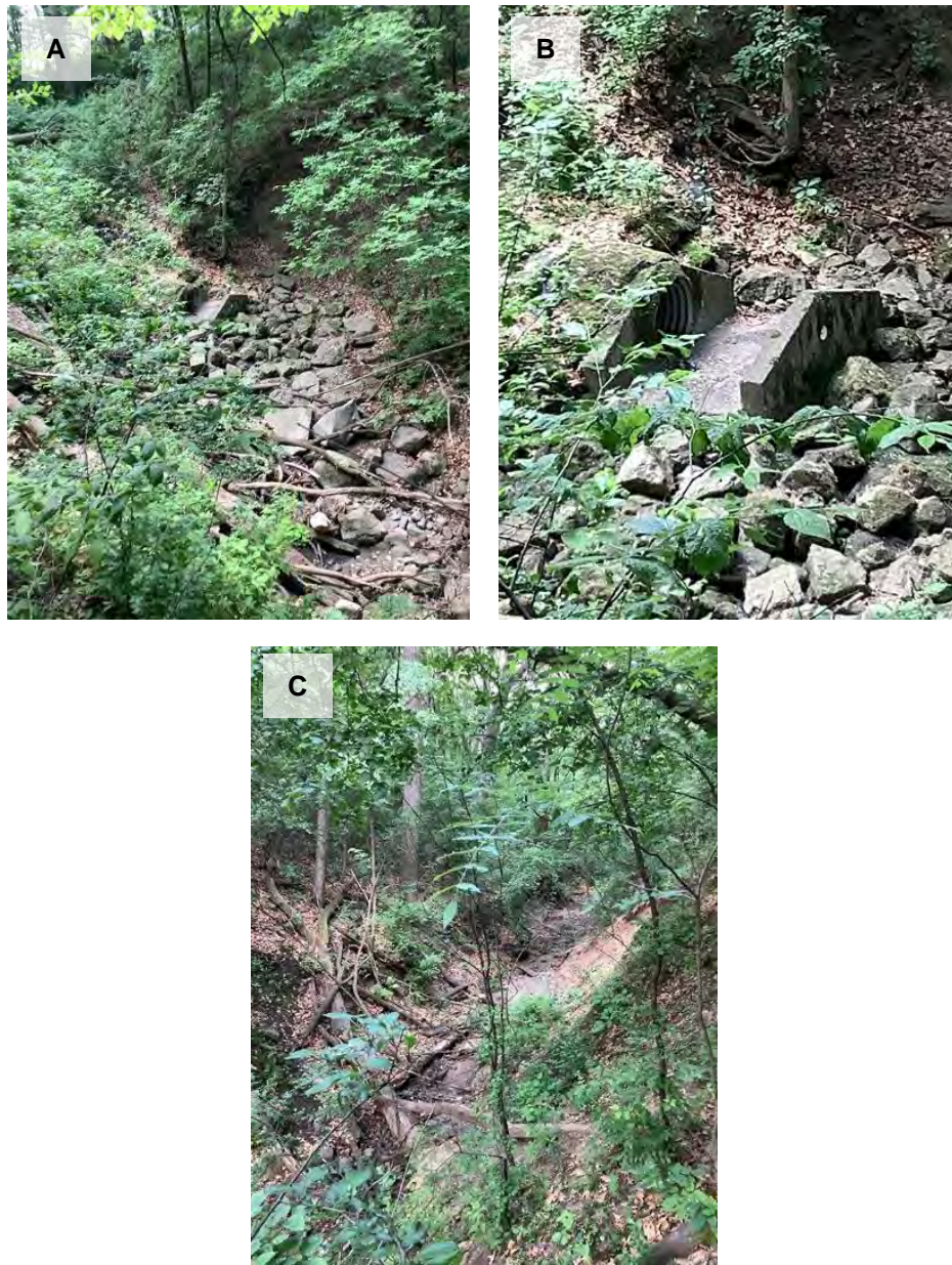
Figure 4: Photos of Gully 06:08-01:06 A) Upstream view of gully, B) Upstream view of pipe, C) Downstream view of gully
