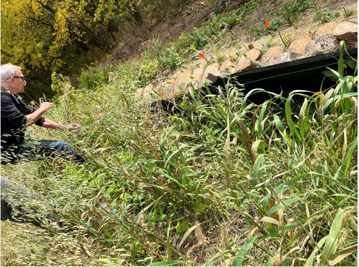
Image 3: Silt fence below Canadian oat cover crop and log berm behind silt fence.
