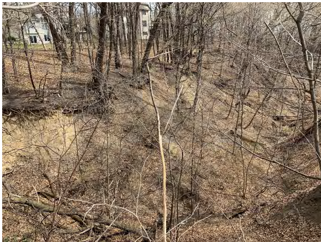
Toe of slope erosion causing slope failure along ravine
