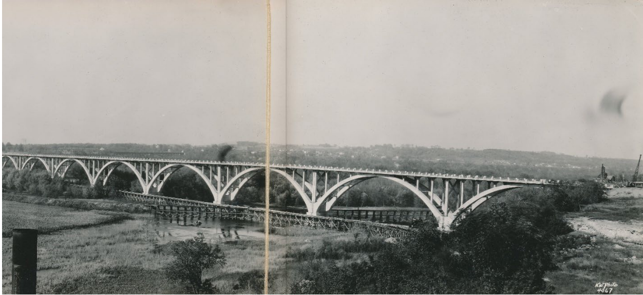
Figure 6. Newly constructed Mendota Bridge in 1926 by the Koss Construction Company from Pilot Knob (Holth 2013)
