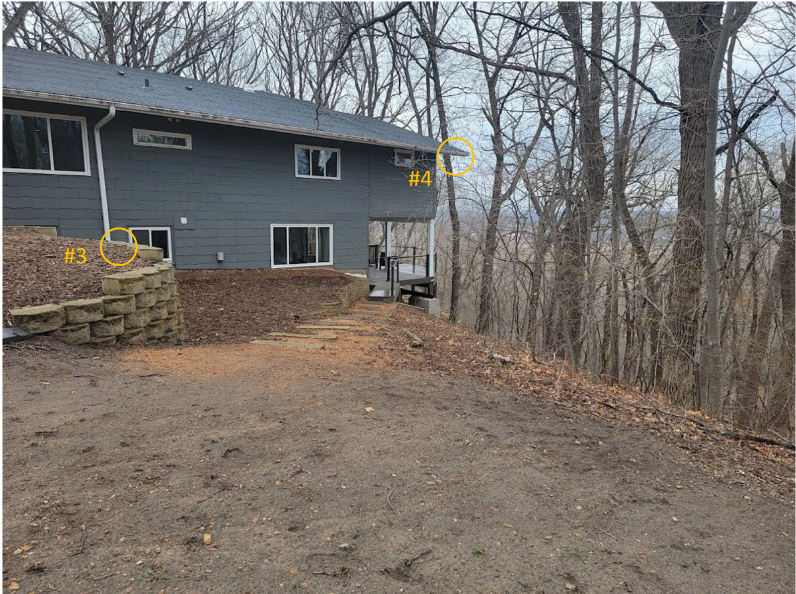
535 Lakota Lane – west side of house (discharge points circled in yellow)
