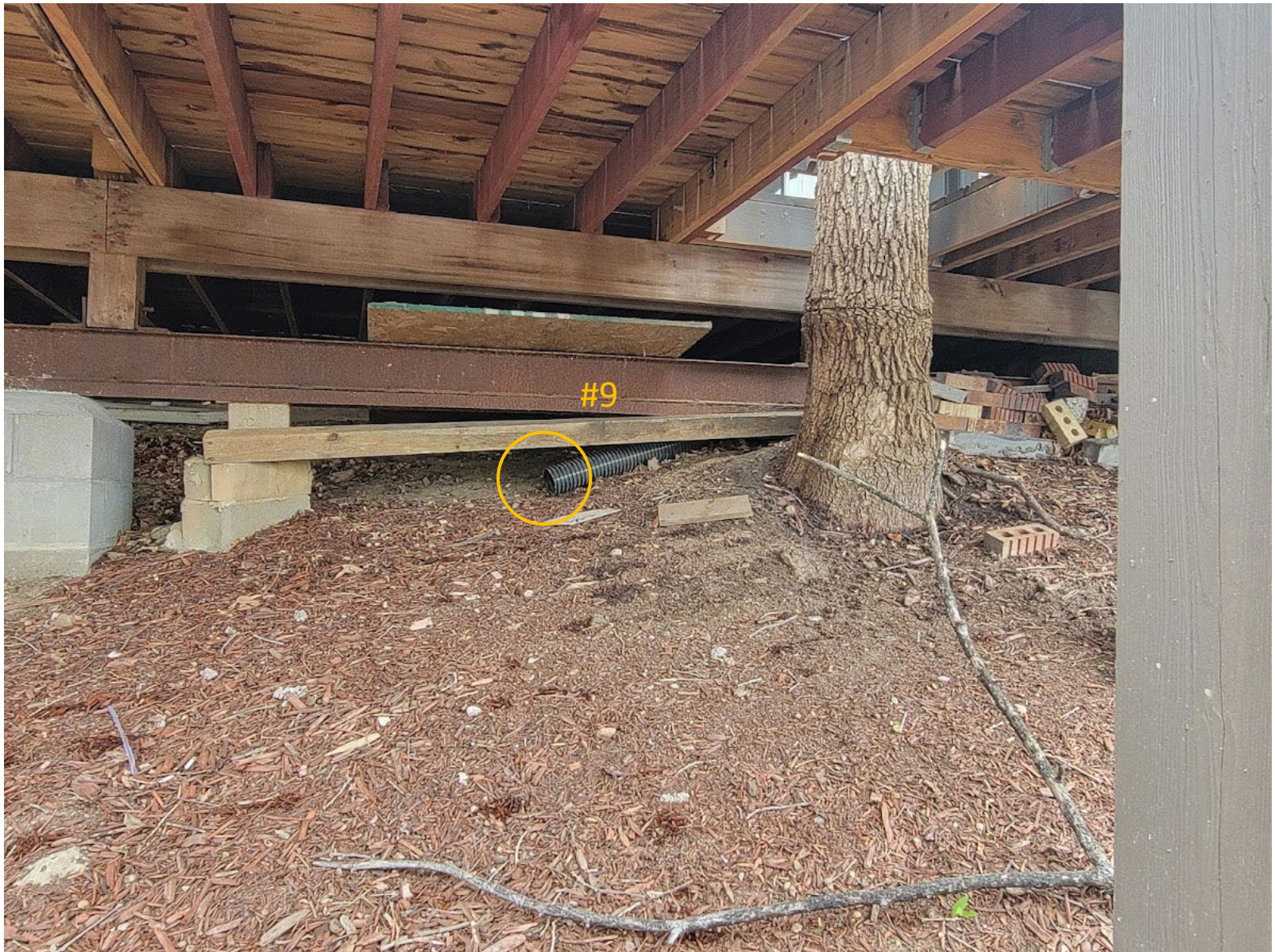
535 Lakota Lane – south side of house, under existing deck
