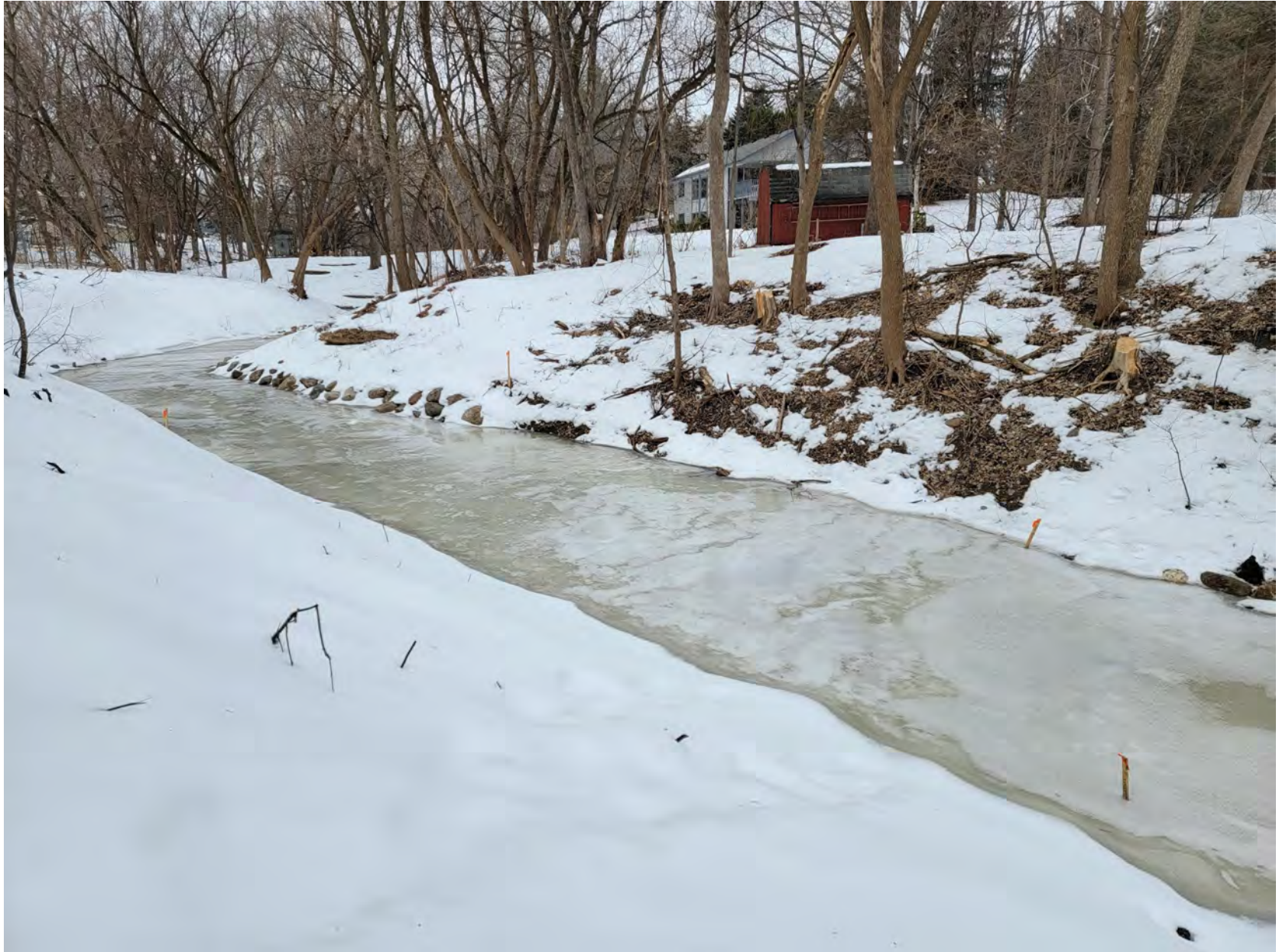
Looking upstream toward start of project from right bank at left bank anchored slope protection (grading, hydroseed and rock toe)
