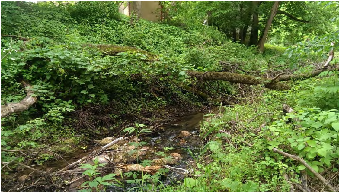
Photo 6: Bank erosion looking towards the residence at 112 5 th Street West. Bank is approximately 40 feet from the structure.
