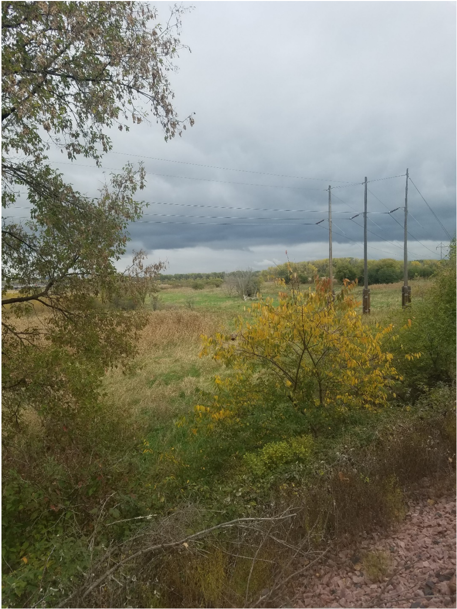
Figure 4. Looking northeast at the Xcel Energy overhead power lines and towers that will be replaced.
