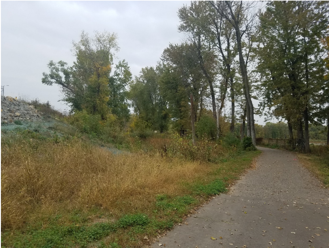
Figure 2. Looking north at the existing trail and I-35W embankment.
