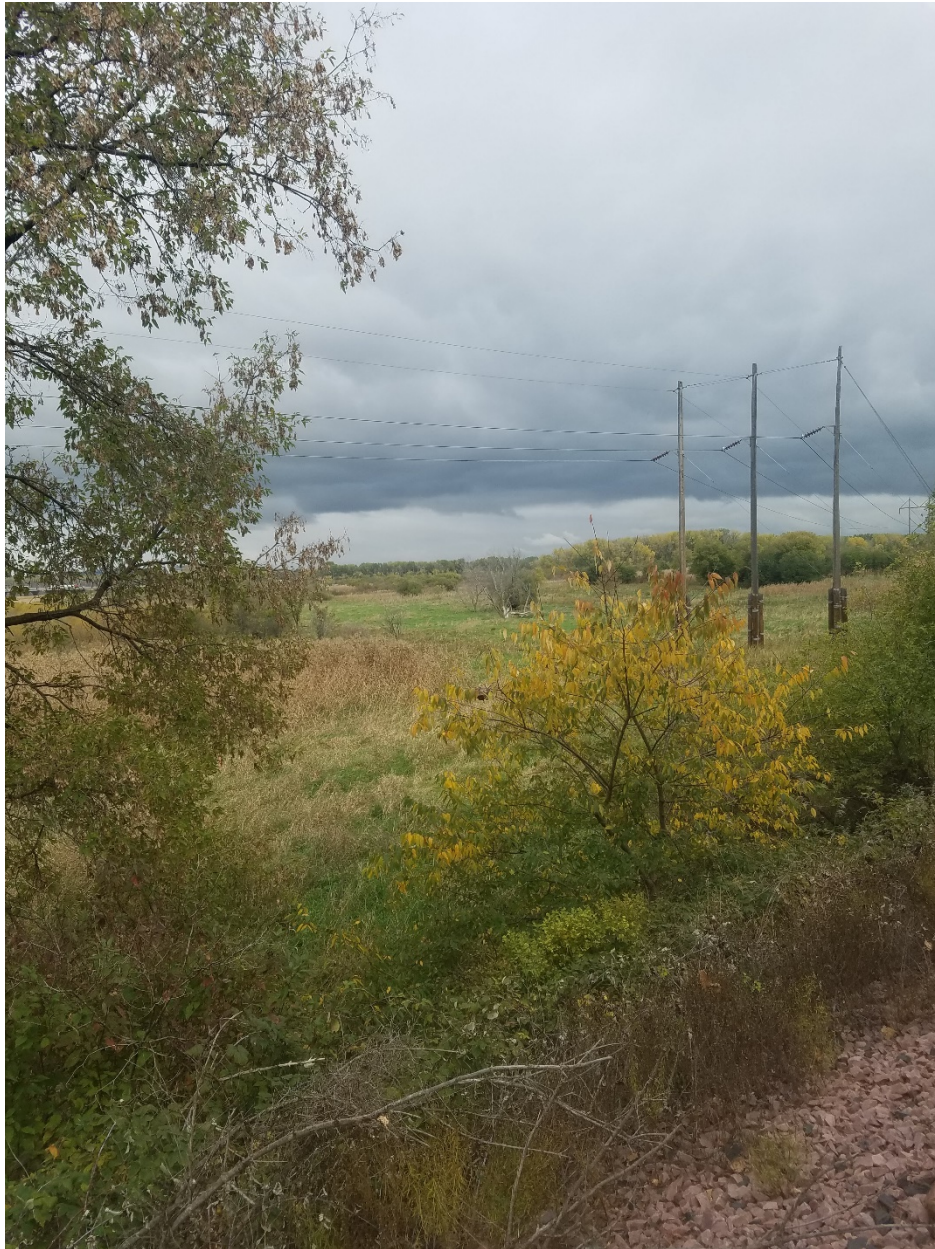
Figure 4. Looking northeast at the Xcel Energy overhead power lines and towers that will be replaced.
