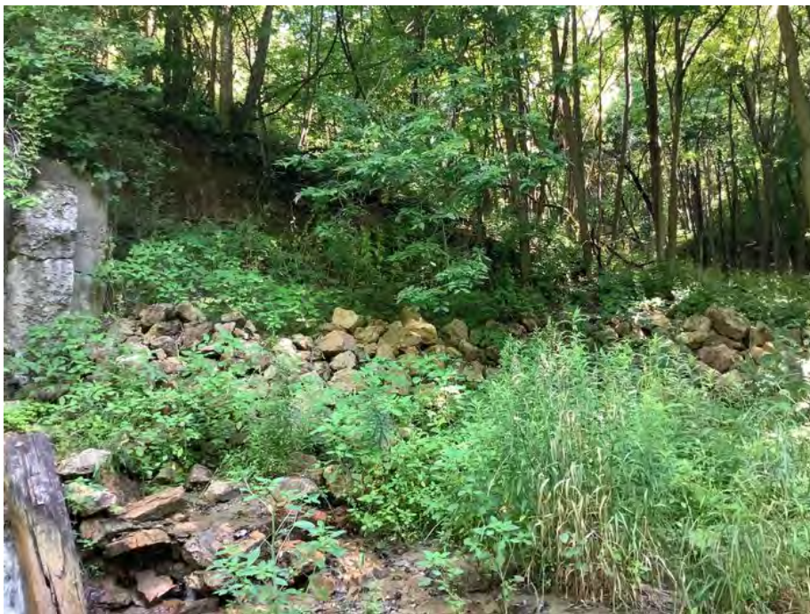
Riprap stabilization along the left bank
