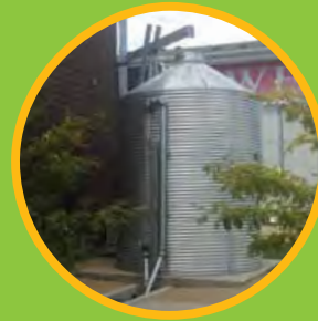
The clear pipe on the front of the cistern shows how much water is inside. Can you tell how full the cistern is today?
