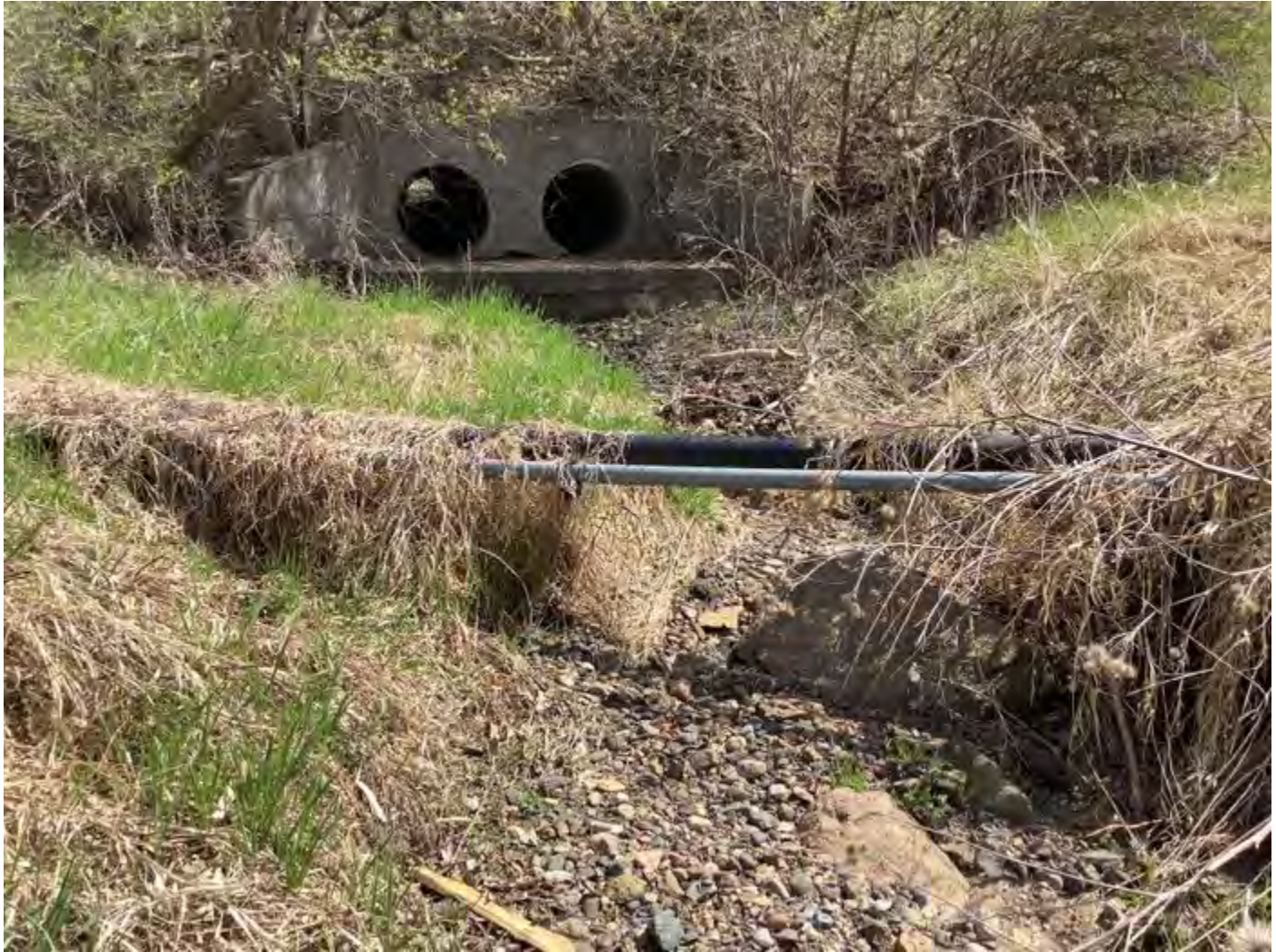
At wetland entrance
