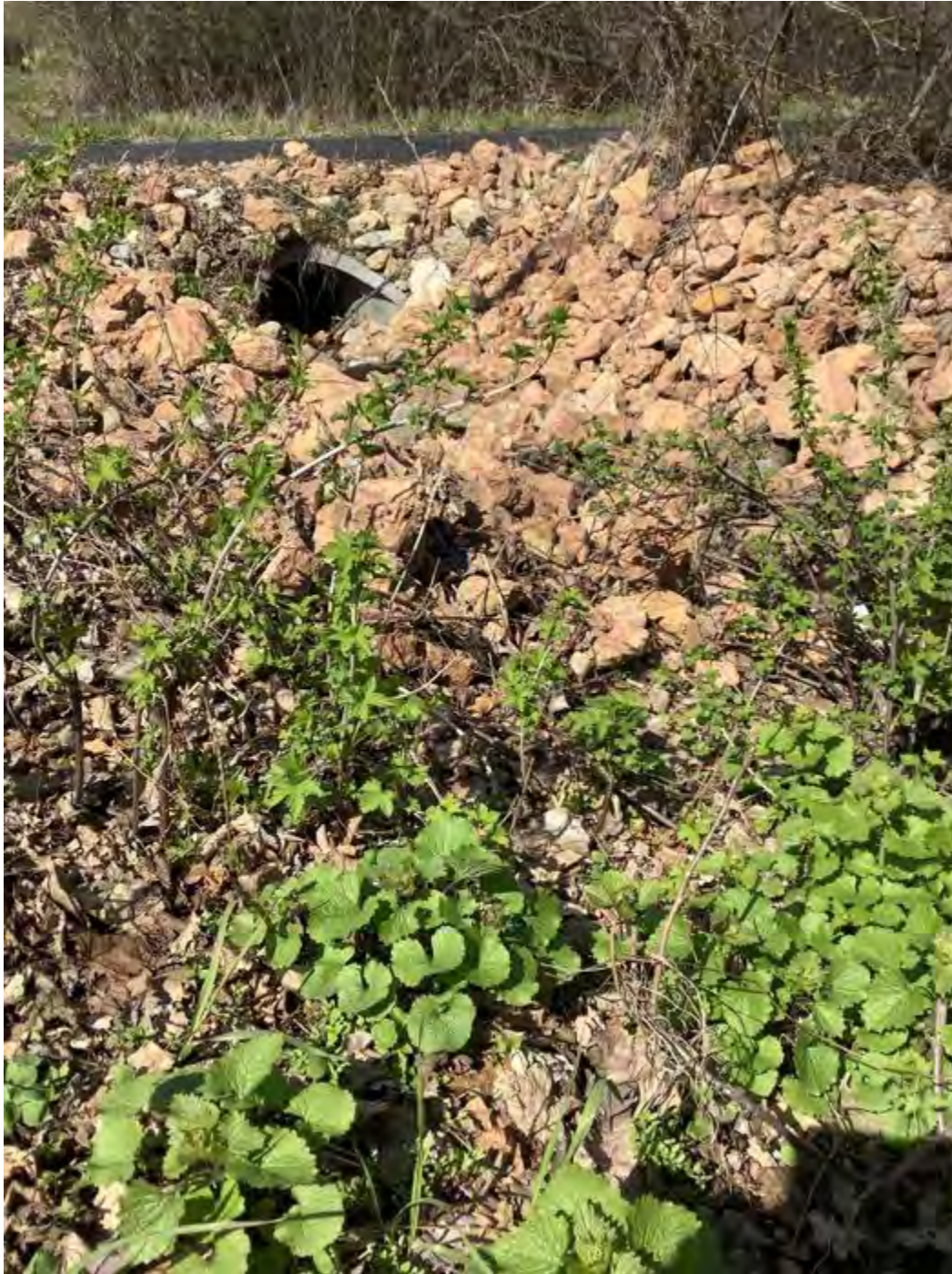
Riprap surrounding outlet feature
