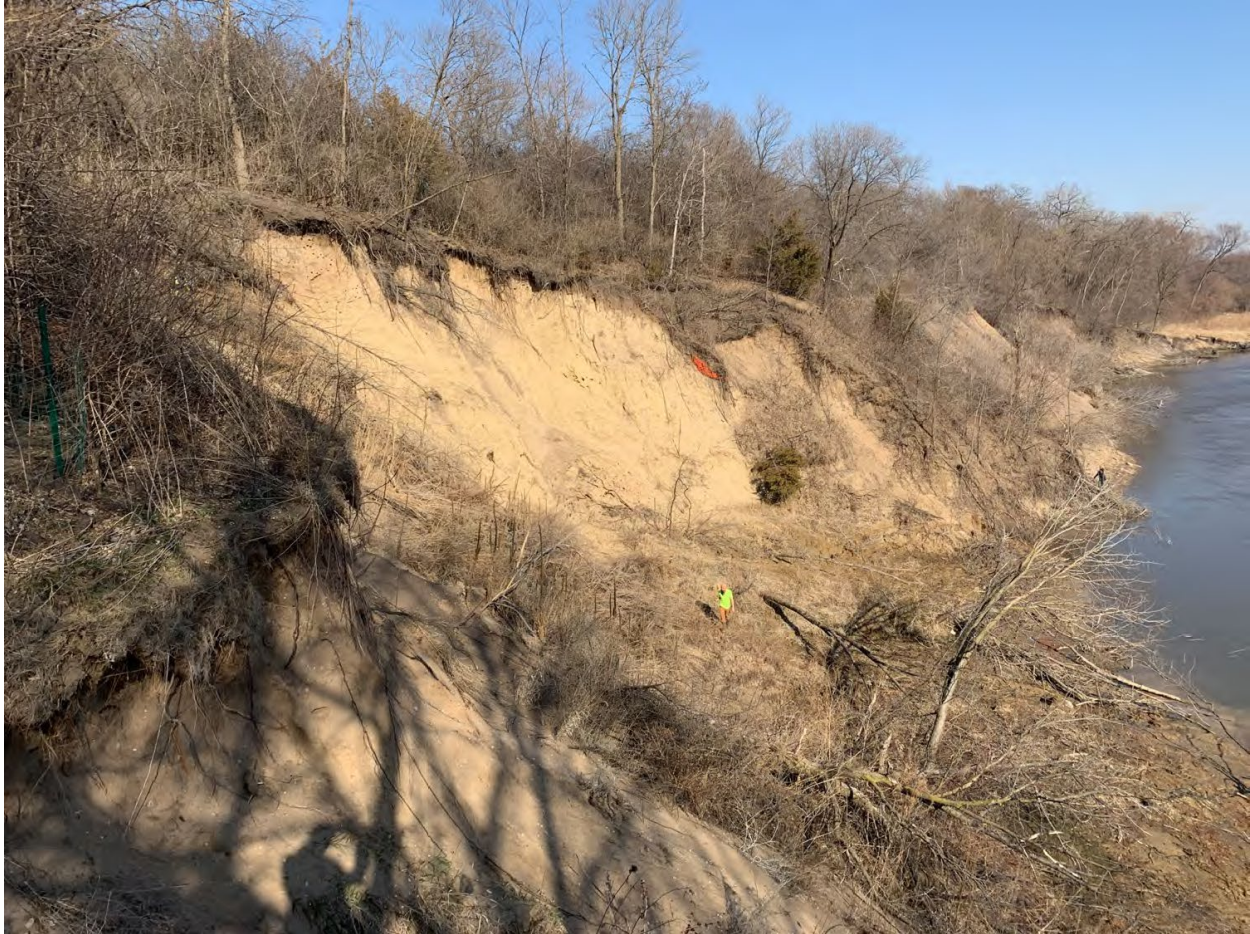
Figure 3. Inter-Fluve site photo looking downstream at Area 3 erosion on May 6, 2021.
