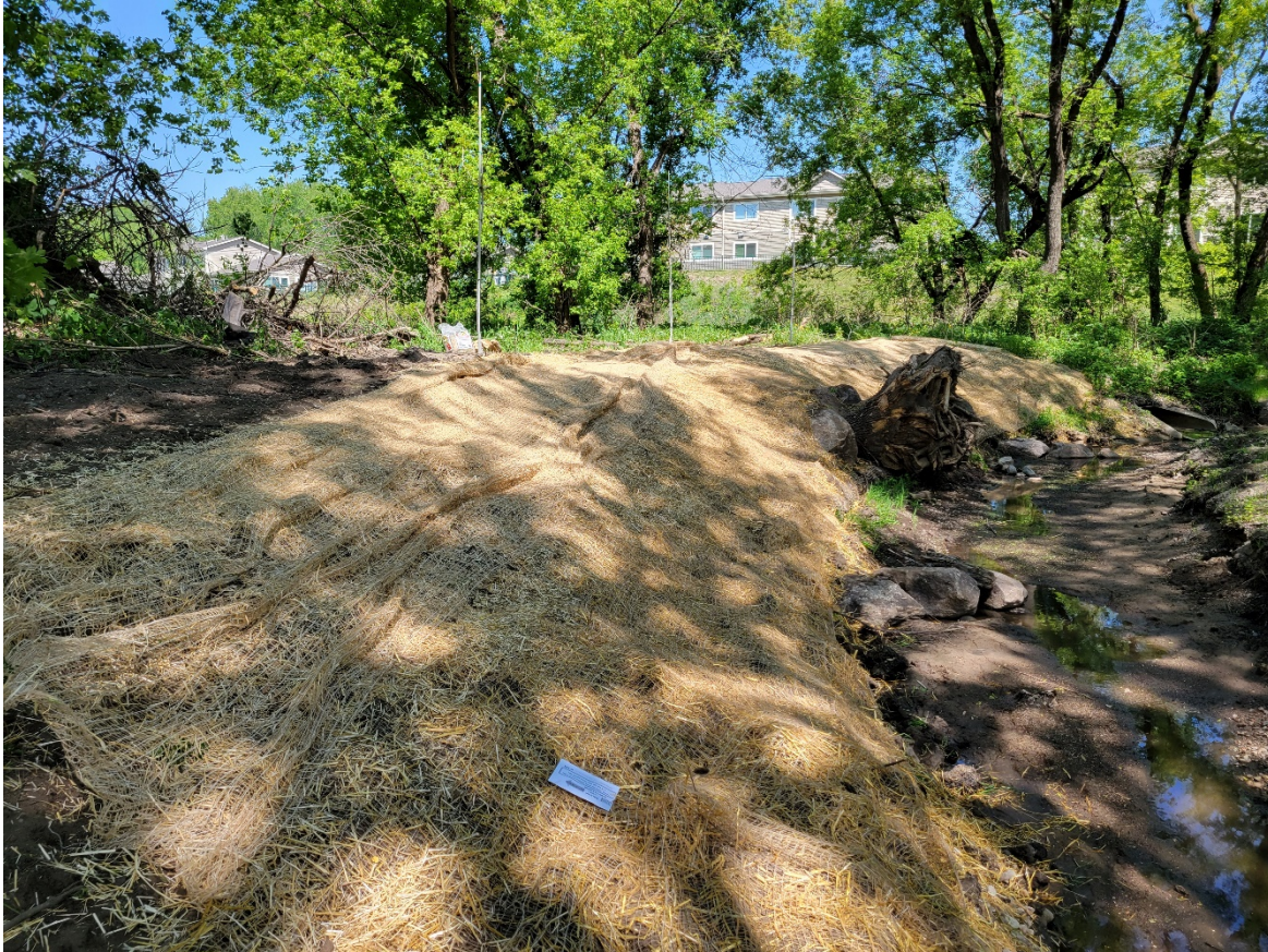
Cut back steep slope near large root wad station 8+30, seeded and added blanket
