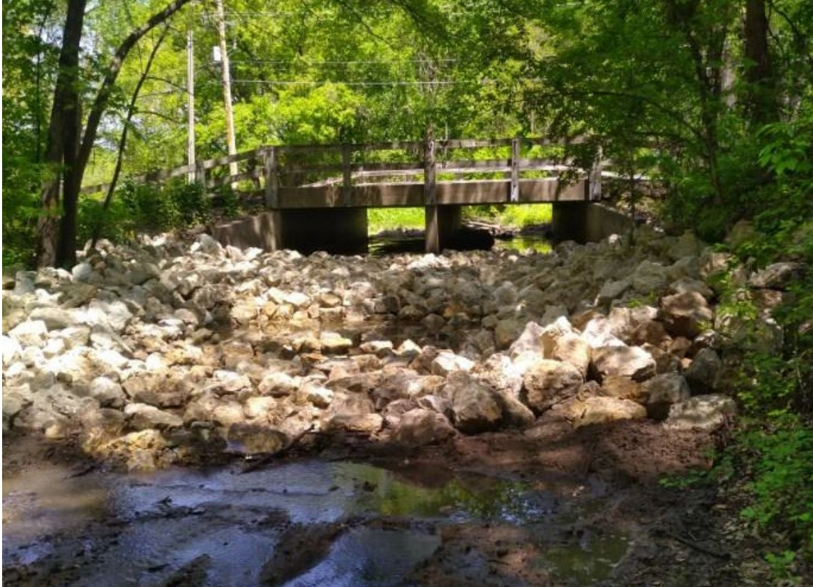
Plunge pool riprap installed, access restored with seed and blanket
