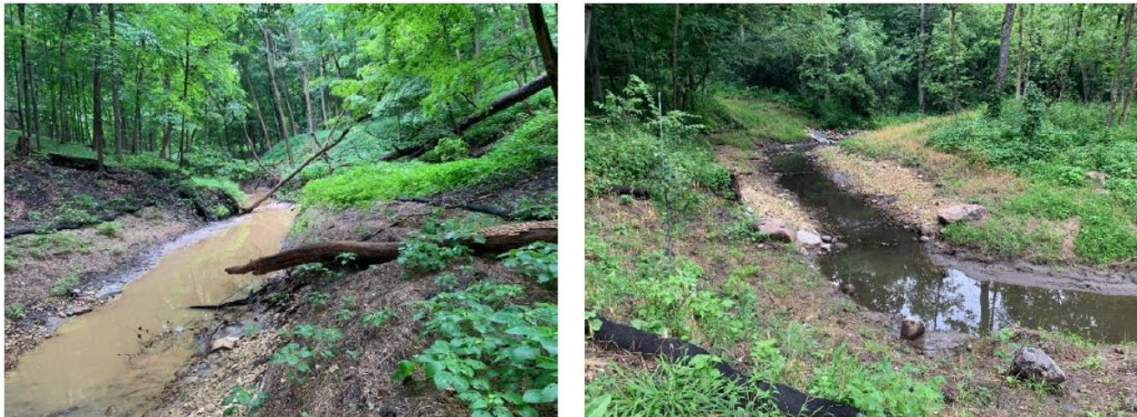
Figure 2. Example of how the restored reach is reducing sediment load downstream; left photo shows streamflow entering the restored reach, and right photo shows streamflow leaving the restored reach downstream (provided by RPBCWD).
