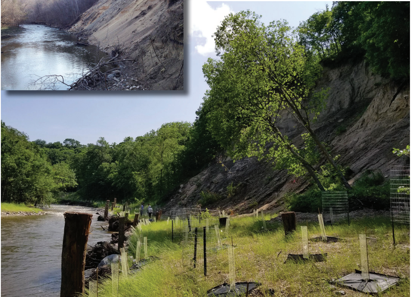
Before and after photos of the Sand Creek Engineered Log Jams Bluff Stabilization in Jordan, MN (2016-2019).
