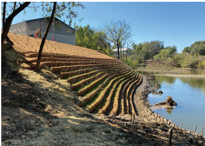
Napa River HDV Bank Stabilization, CA
