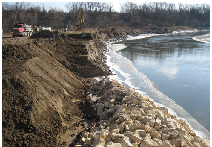
Winter Construction on the Minnesota River.
