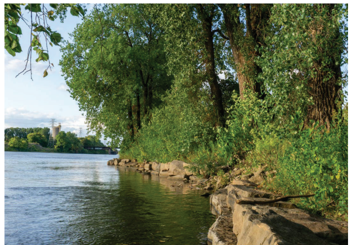
Mississippi River, Sheridan Park Bank Stabilization, MN
