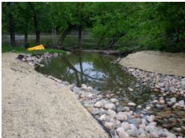
Looking North toward MN River
