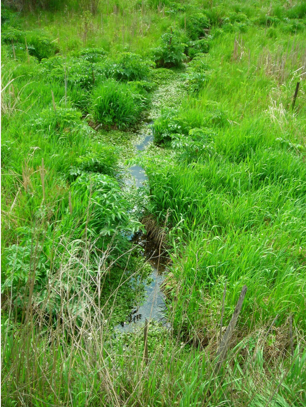
View upstream from R.R. culvert
