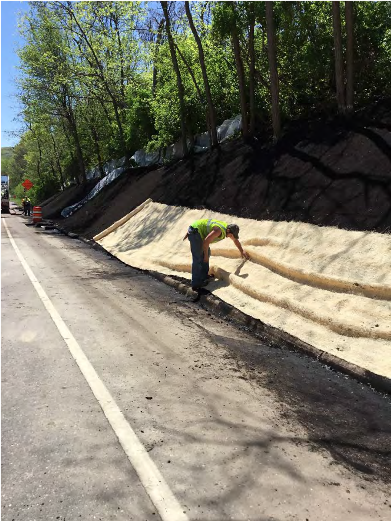
TH 95: Second step of installation/turf establishment (5/12/2017).
