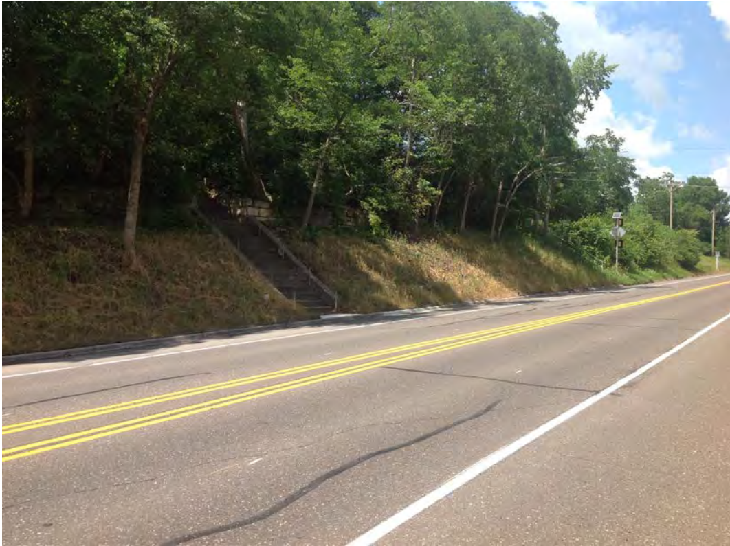
TH95: Inspection 8/4/2017 shows successful turf establishment.
