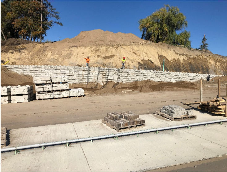
Retaining wall construction along Highway 101
