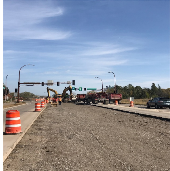
Construction on Highway 61 at the old Highway 101 intersection
