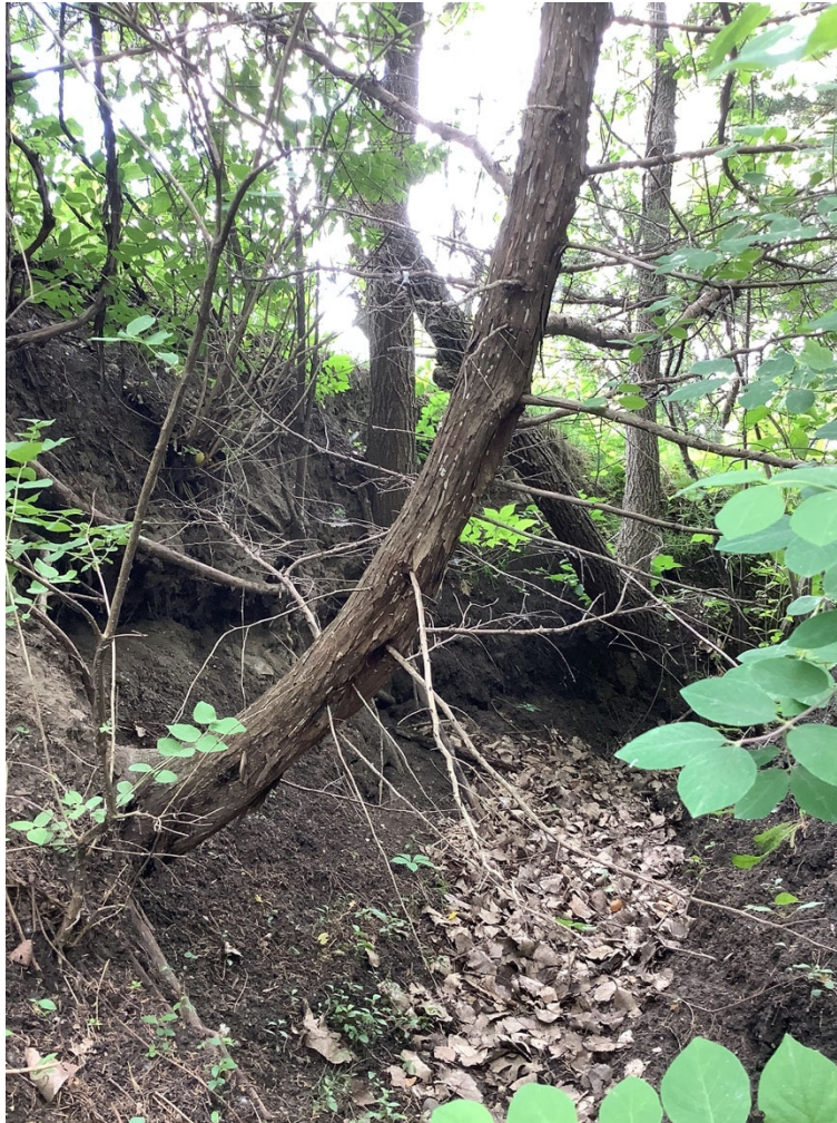
Figure 88. Downstream view of 999-035's channel taken in 2020.
