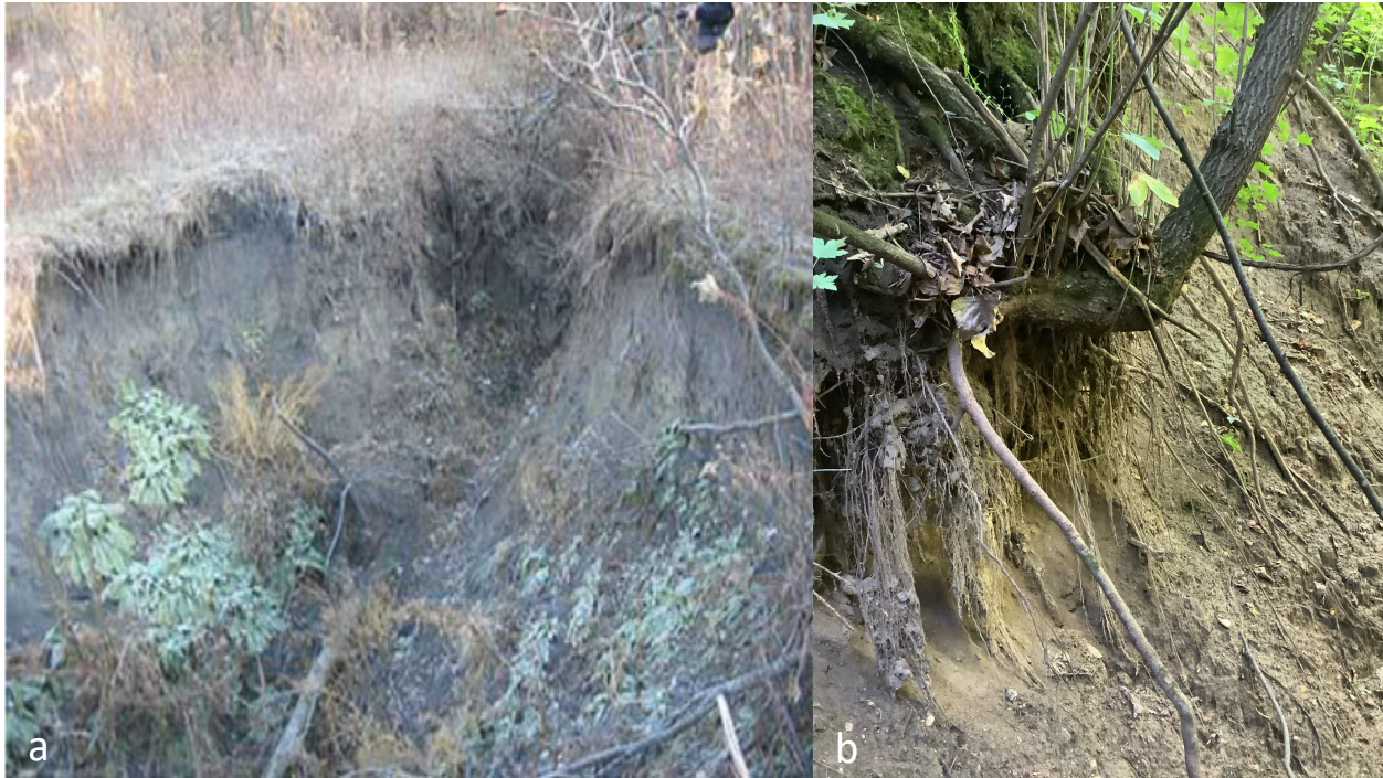
Figure 76. Similar characteristics and active erosion around Gully L203 in 2008 (a) and 2020 (b). Deep incision not seen at time of the visit, possibly blocked by vegetation.
