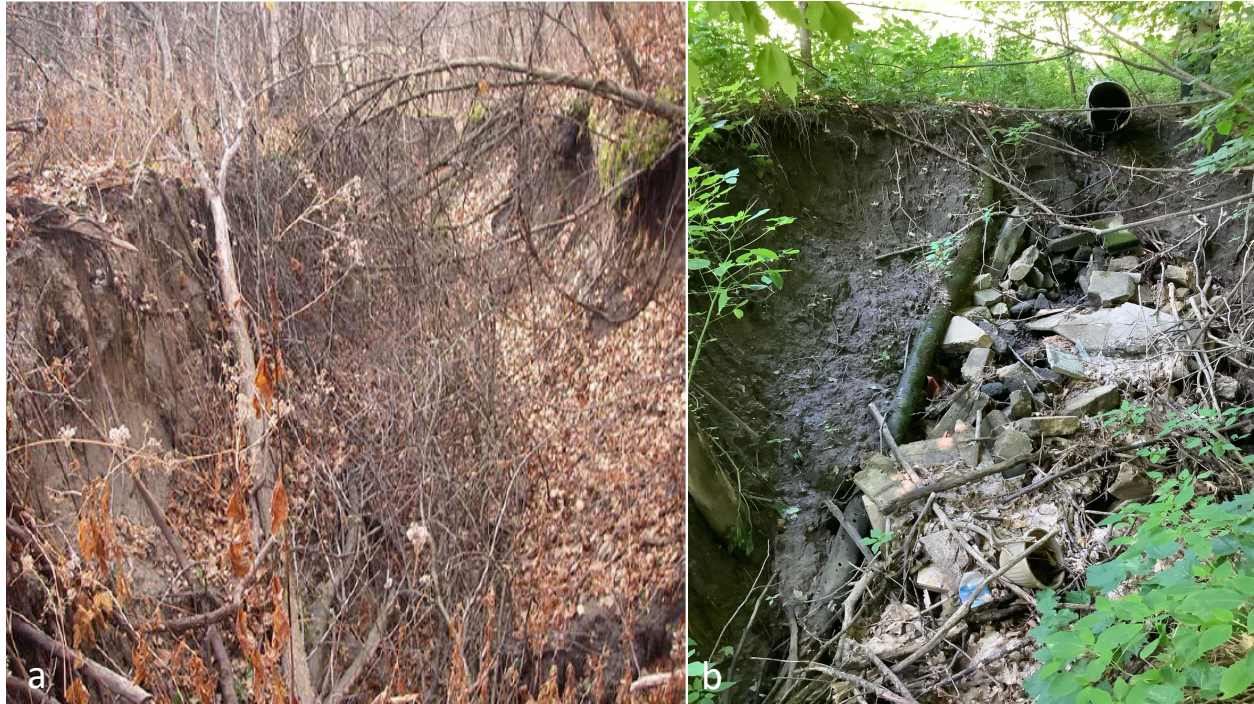
Figure 74. Comparison of gully sites between 2008 (a) and 2020 (b). The 2008 picture shows an unspecified angle of the gully. The 2020 picture shows an upstream view toward the head cut and unstable pipe outlet.
