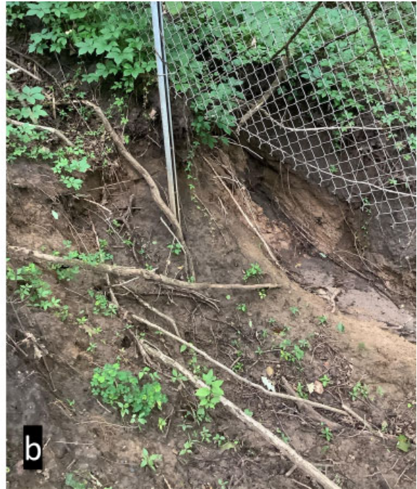
Figure 22. Severe erosion at Gully 999-117. Photo 'a' was taken looking downstream at the head cut. Photo 'b' was taken looking downstream at an incised section of the gully.
