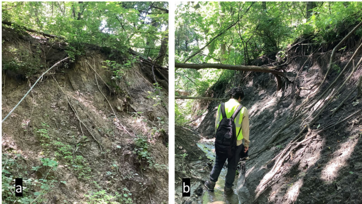
Figure 17. Photos from the 2020 field survey to L219. Person for scale in 'b' emphasizes depth of incision.
