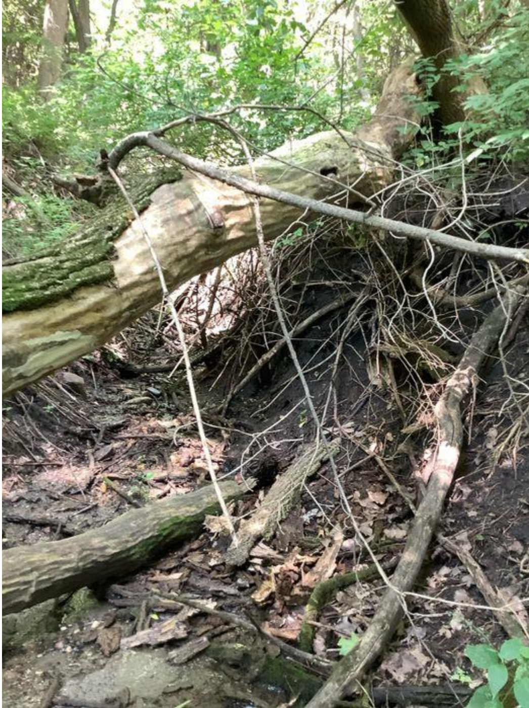
Upstream view of slumping along left bank and channel incision. View from gully bottom near toe.
