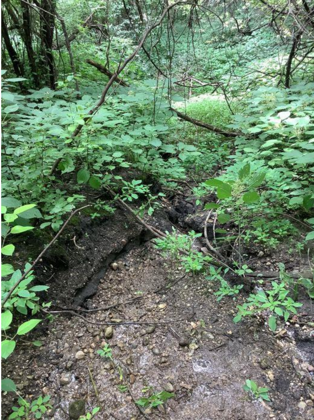
Looking d/s from groundwater seep at headcut and channel incision
