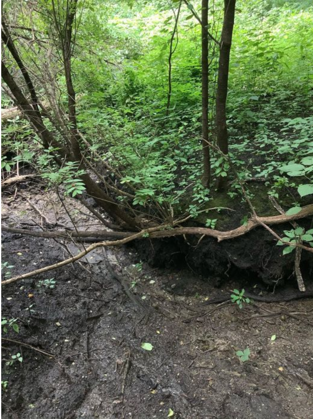
Side stream view from left bank looking at section of overhang on right bank.
