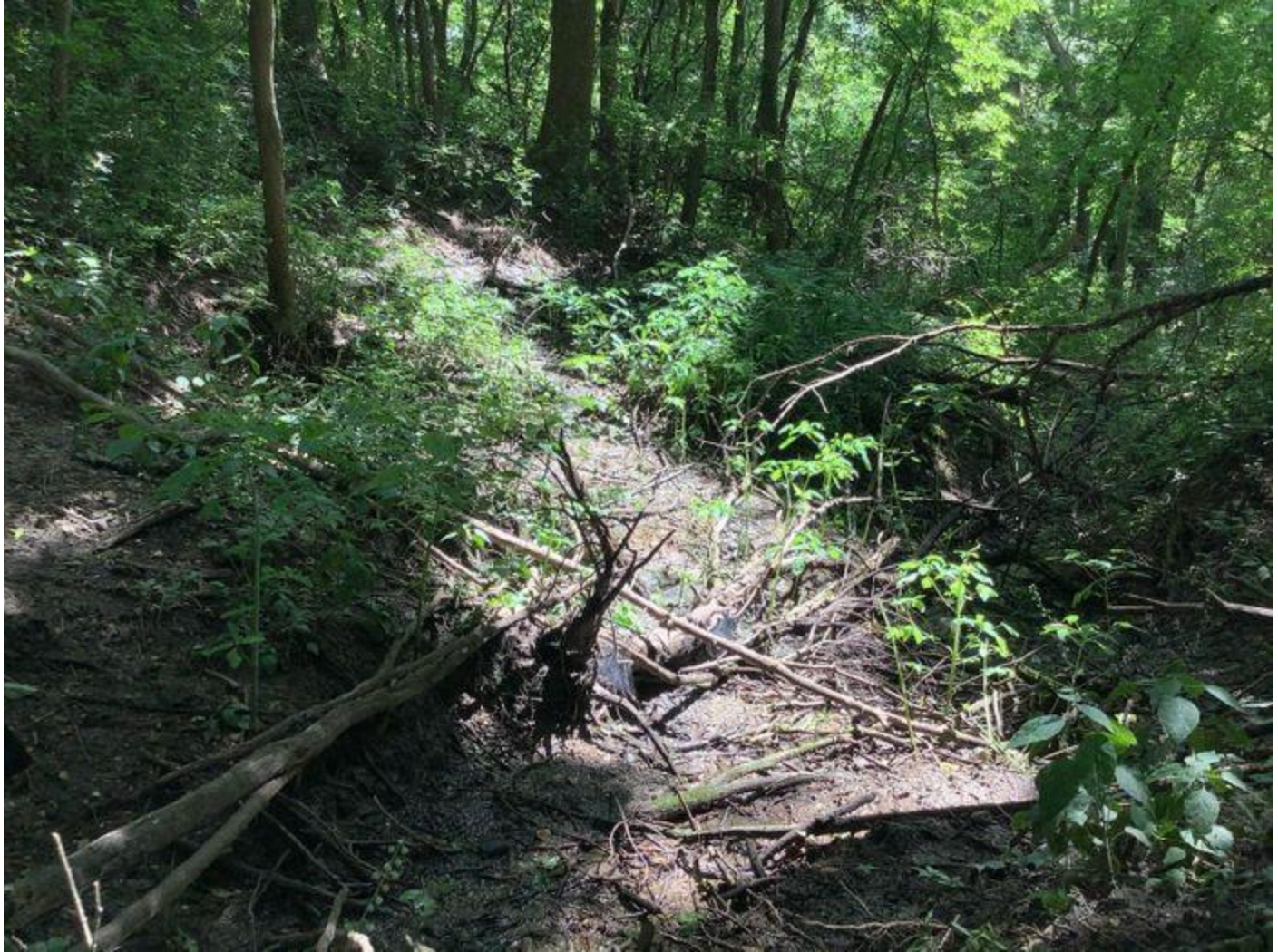
Downstream view from right bank of headcut looking at large slump along left bank.
