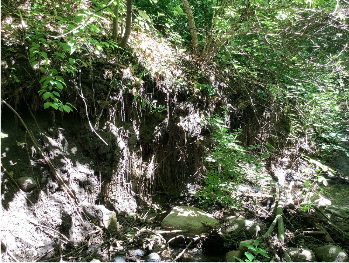
Figure 6. Looking downstream at left bank overhang.
