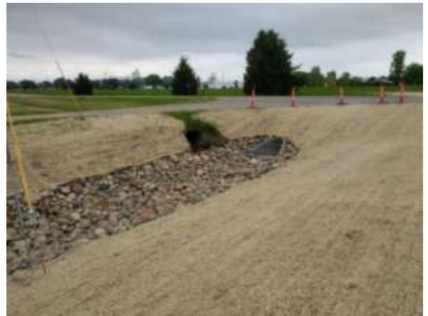
Drainage outfall - looking southeast
