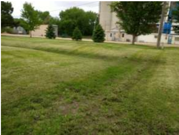
Drainage to pipe under service road to back of Riverland elevator - from frontage road
