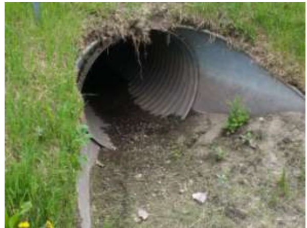
End of pipe under frontage road
