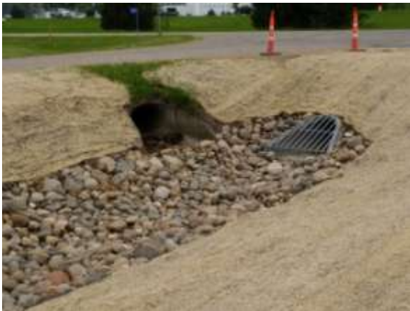
Drainage outfall - looking southeast
