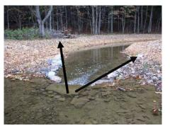
Riprap Toe Protection Rock riprap placed along the streambank to dissipate energy, protecting the slopes from erosion
