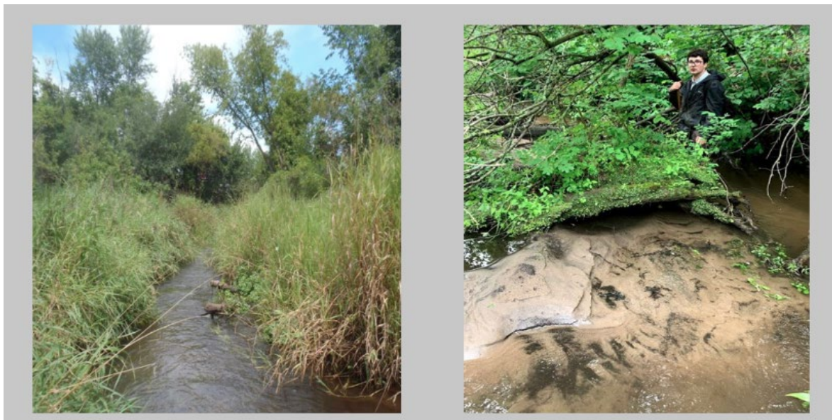
Figure A.2. Eagle Creek in 2014 on left and picture of increased aggradation in 2019 on right. Brenda DeZiel (2014). Kirsten Haus (June 2019).
