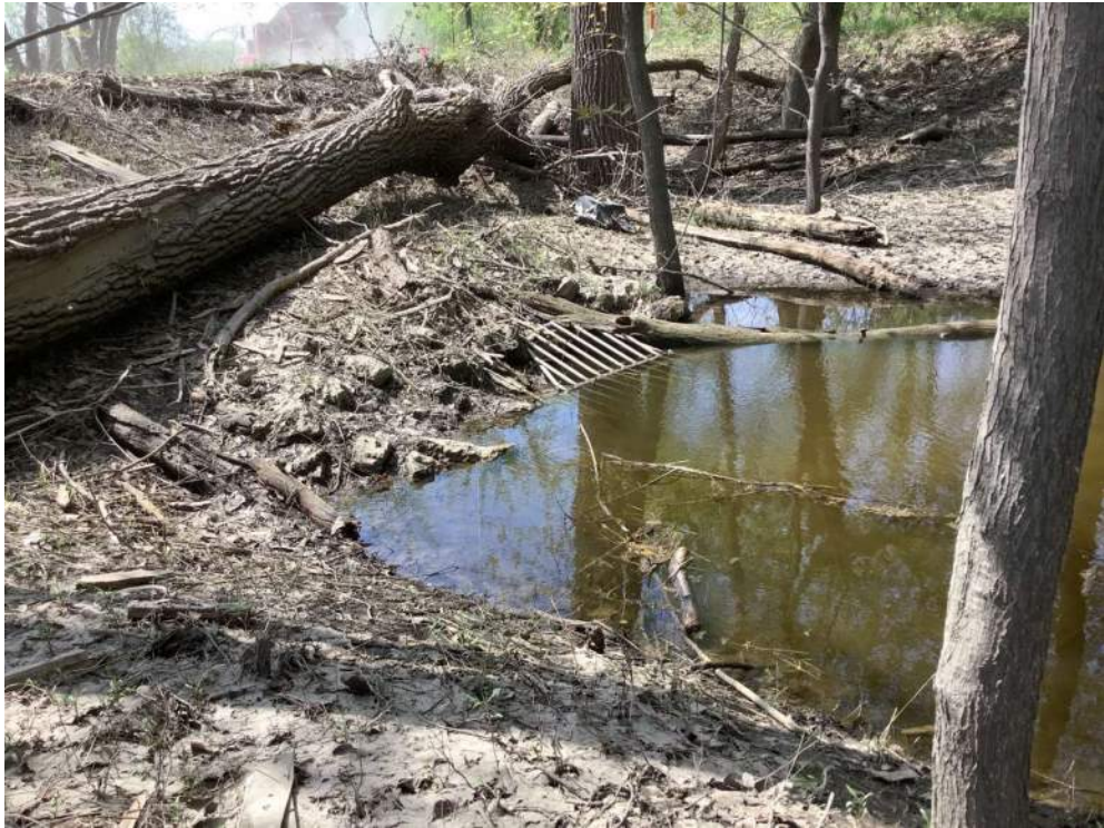
Photo 3 – View of a culvert connecting Wetlands A1 & A3, facing south.
