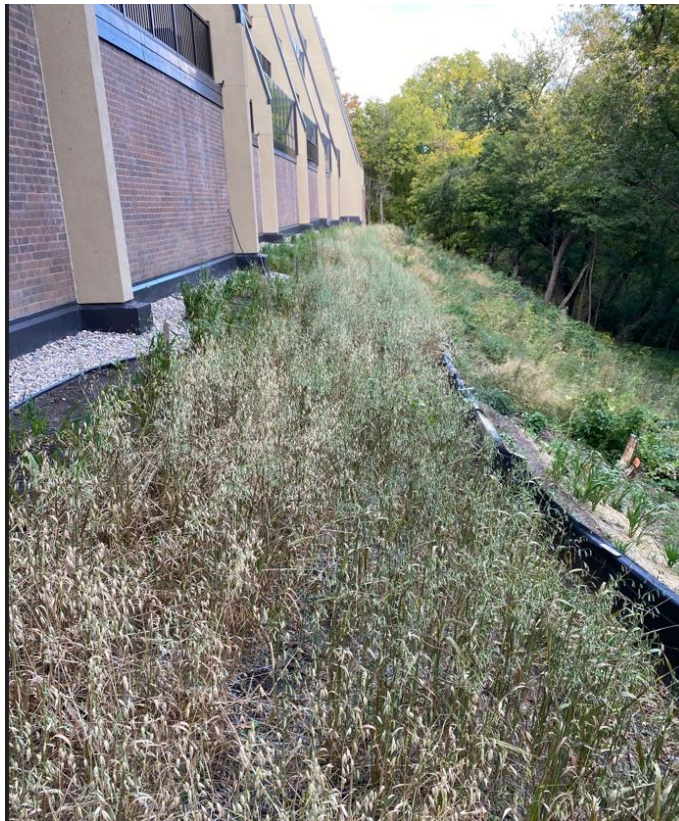
FIGURE 1. October 02, 2022 Looking east. Canadian Wild Oats nurse crop for the Mesic Prairie SW seed. Rock covering drain tile is visible near building. Silt fence was removed except for top of 2 test areas.
