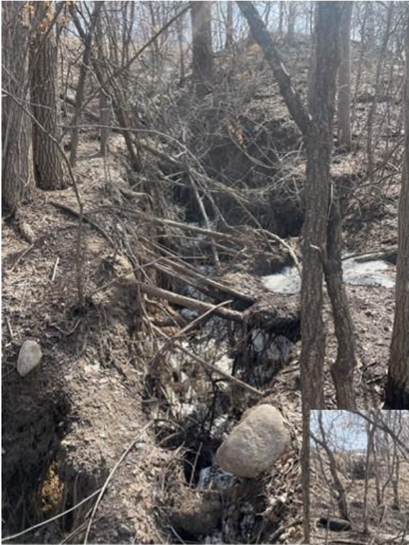
Attachment 2— Ravine Stabilization Site existing conditions photos
