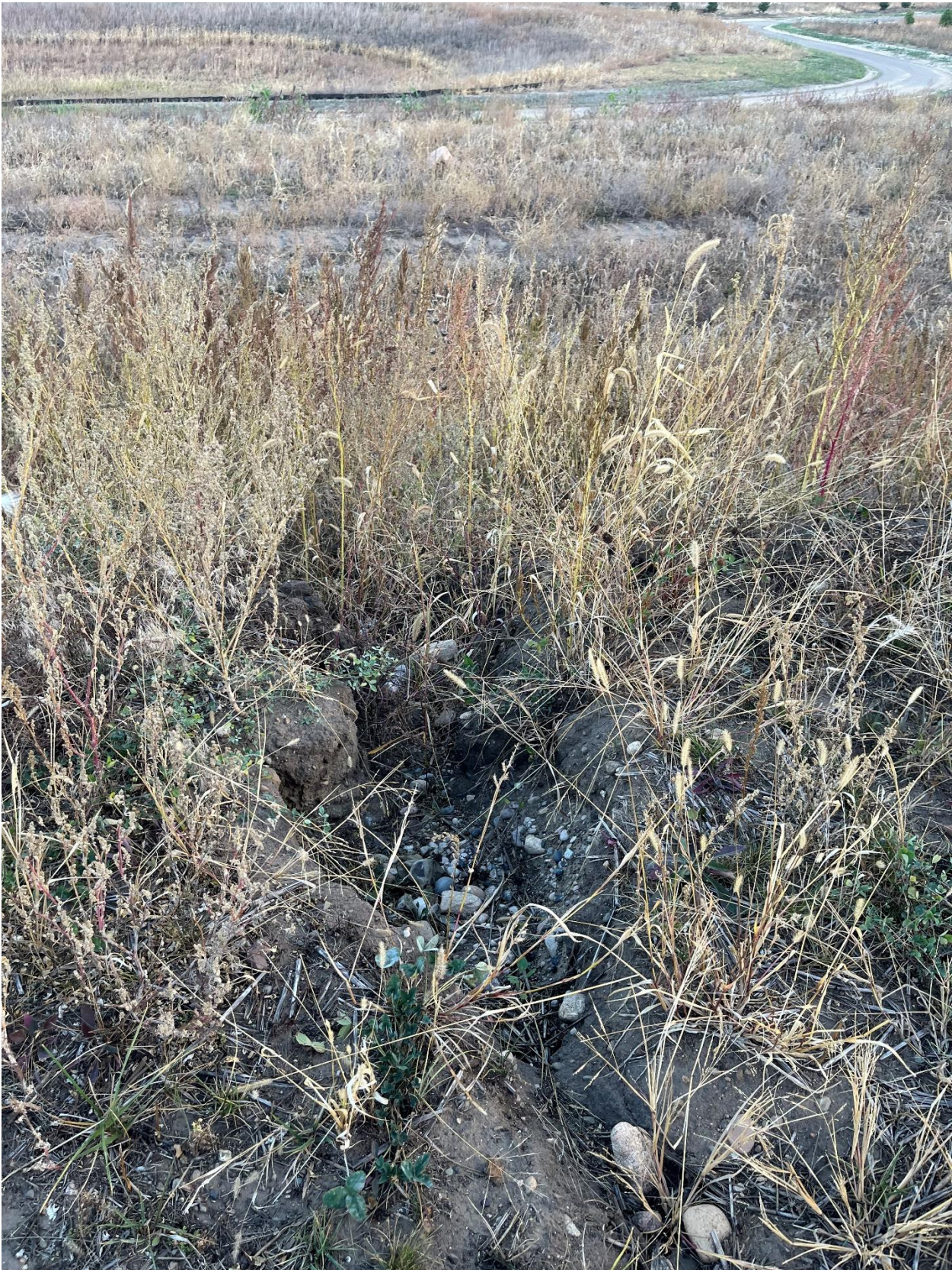
Figure 8. Remaining Erosion North of Tyrone Drive 10/12/2022
