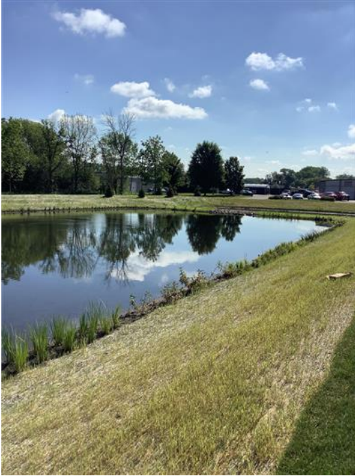
Figure 4. Erosion control blankets surrounding pond
