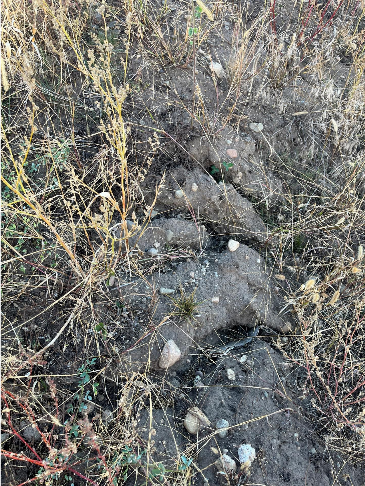
Figure 7. Remaining Erosion North of Tyrone Drive 10/12/2022
