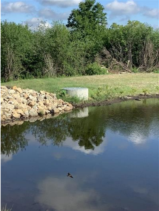
Figure 3. Western emergency overflow
